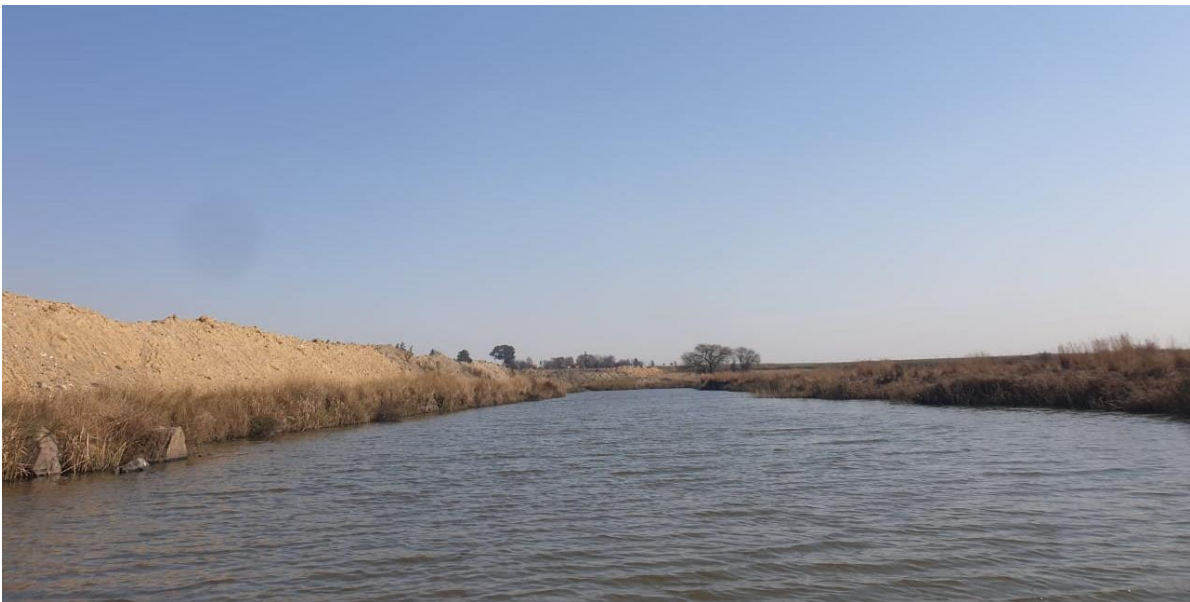
FIGURE 15: OLIFANTS RIVER- NOTE EMBANKMENT ON THE LEFT OF THE IMAGE
