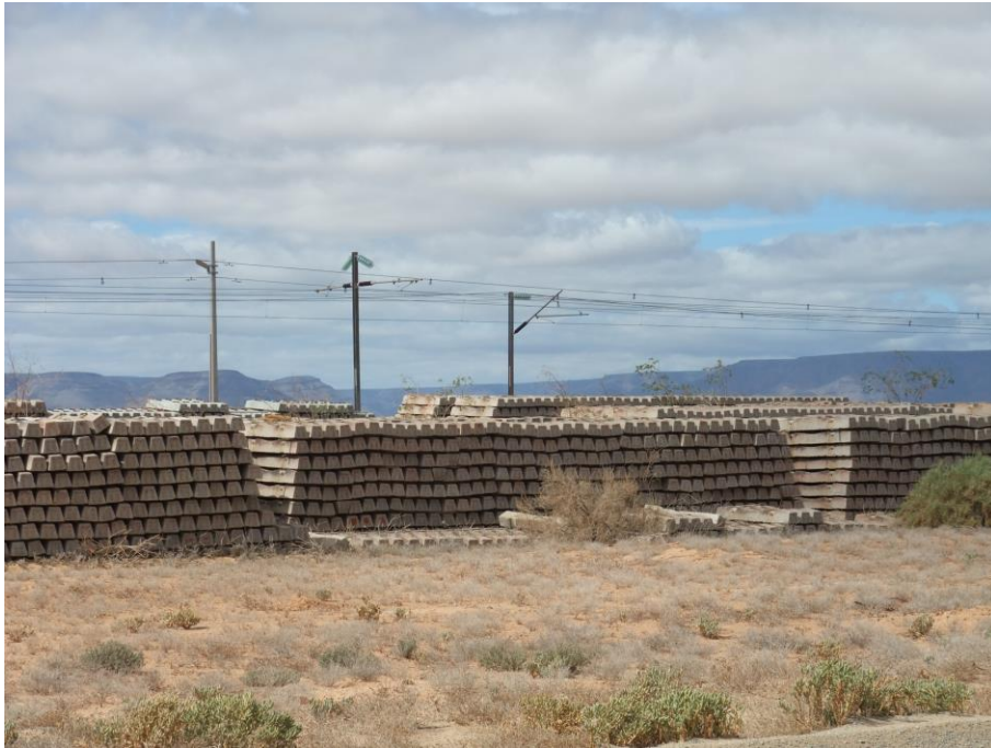
FIGURE 11: THE RAILWAY LINE ON THE FARM. IT CURRENTLY IS UNDERGOING MAINTENANCE.
