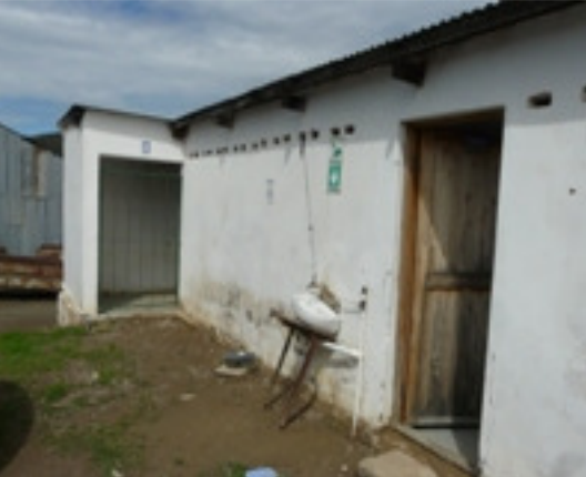
S2 – Ablution facility
