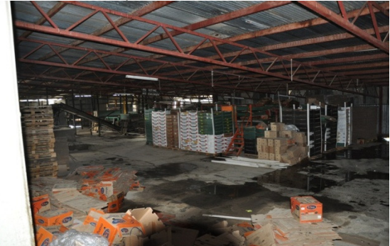
S2 – Internal view
