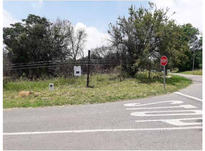
View of the site from Spruce Street
