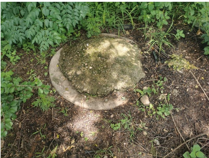
Manhole observed on site
