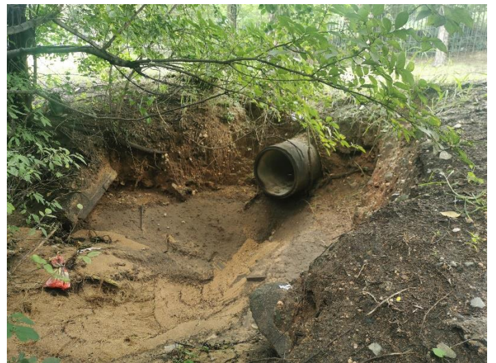
Stormwater pipe discharges into the site
