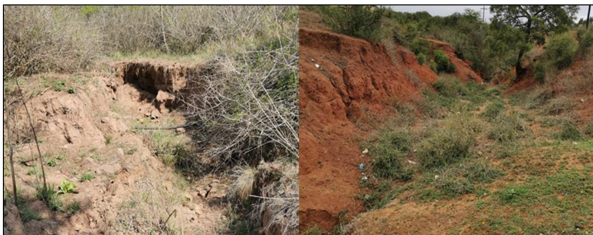
Figure 31: Examples of erosion seen within drainage lines (November 2019)
