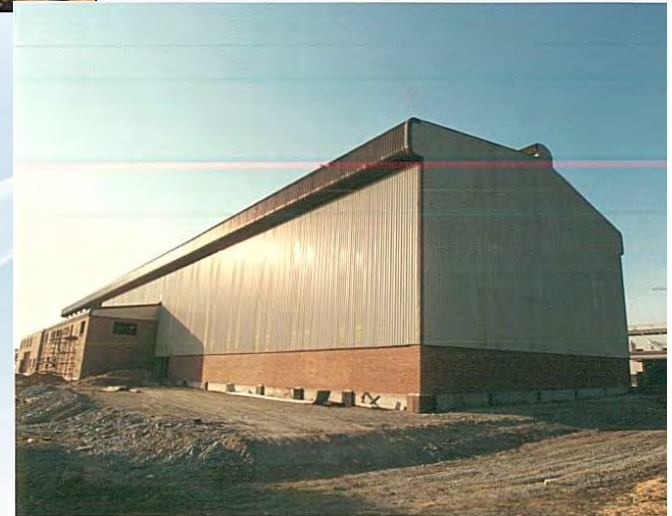
Base metal refinery – the hydrometallurgical plant at PPM will be a similar installation
