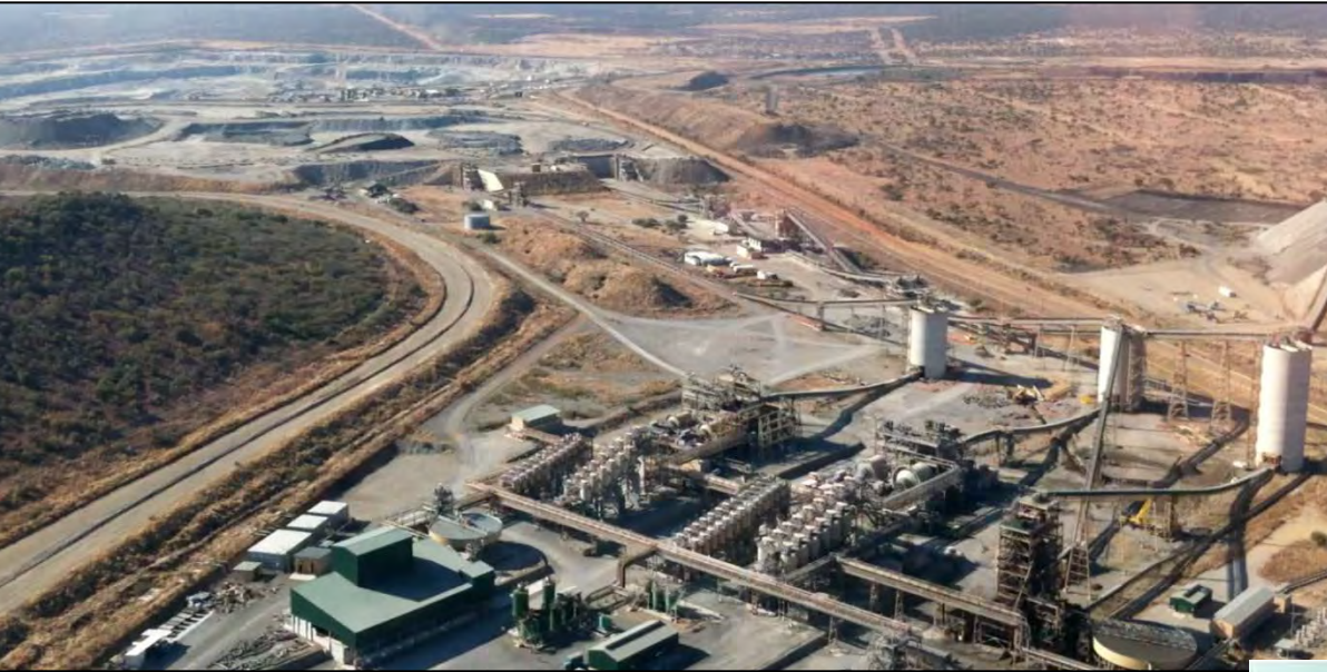
Existing PPM Plant
