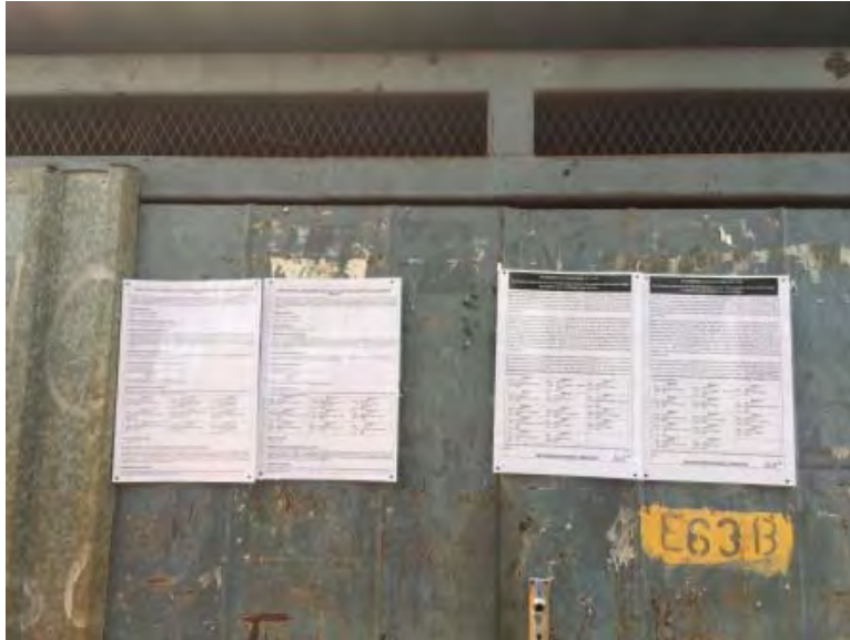
Water Pump - Magalane
