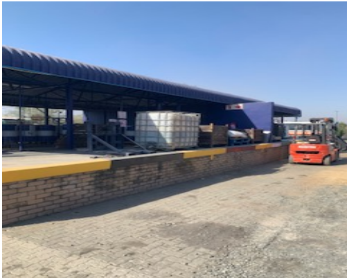
13. Infrastructure middle of northern site. View N
