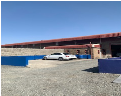
10. Existing infrastructure on the site. View E
