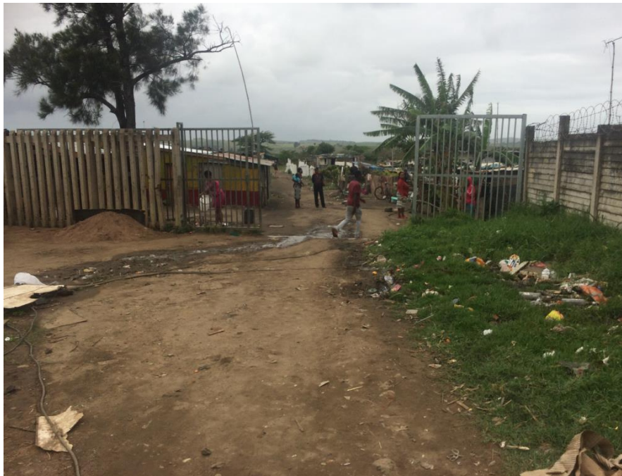
Figure 2: View towards the site gate
