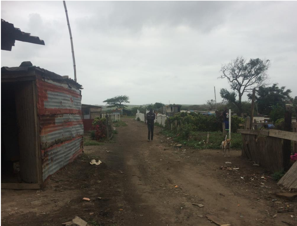
Figure 5: Main access road within the landfill boundaries
