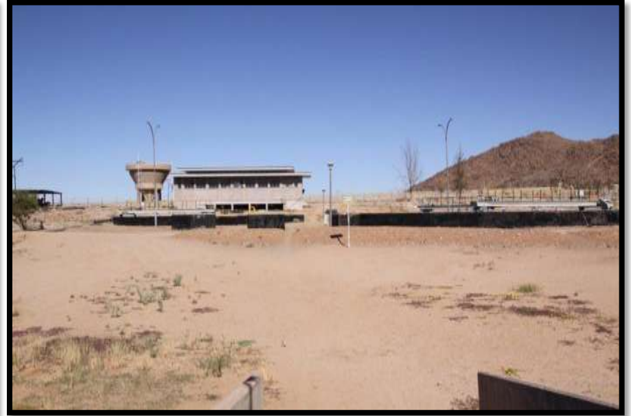
Henkries water treatment works and clear water pumpstation (WTW)
