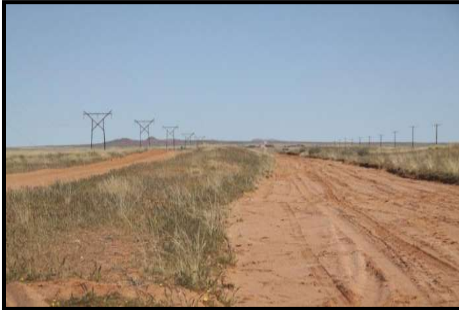
Between Henkries WTW and Doornwater booster pump station (N-S)
