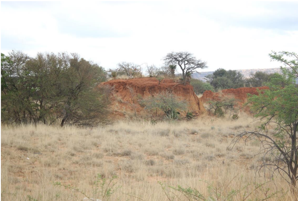
Figure 8: View of some of the dongas located North West of the waste body within the landfill boundaries
