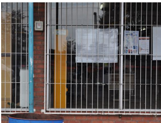
Site Notice 1: Black Rock Supermarket
