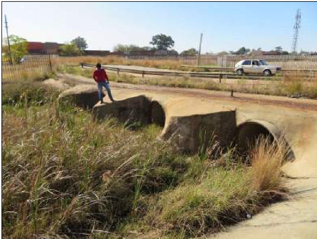
Figure 7-1 Heine Miller street culvert
