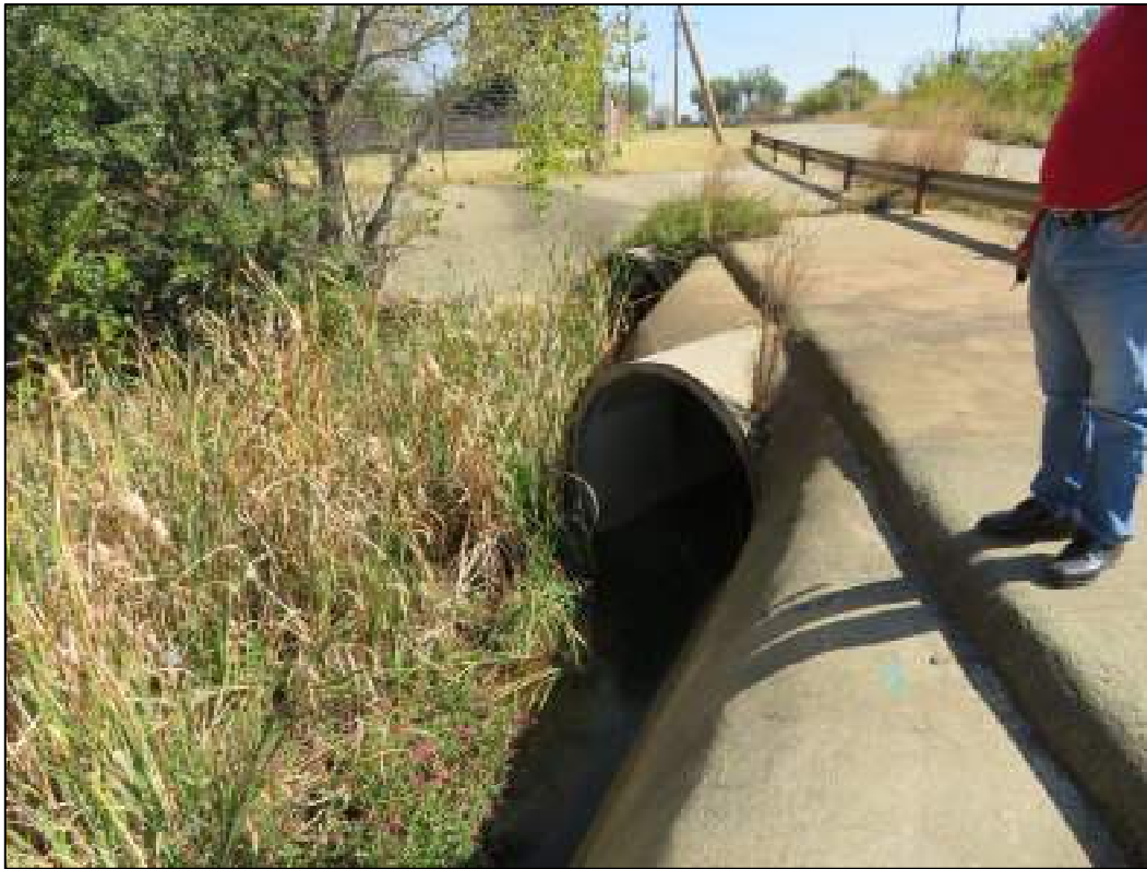
Figure 7-2 Doodles Tapscott street culvert
