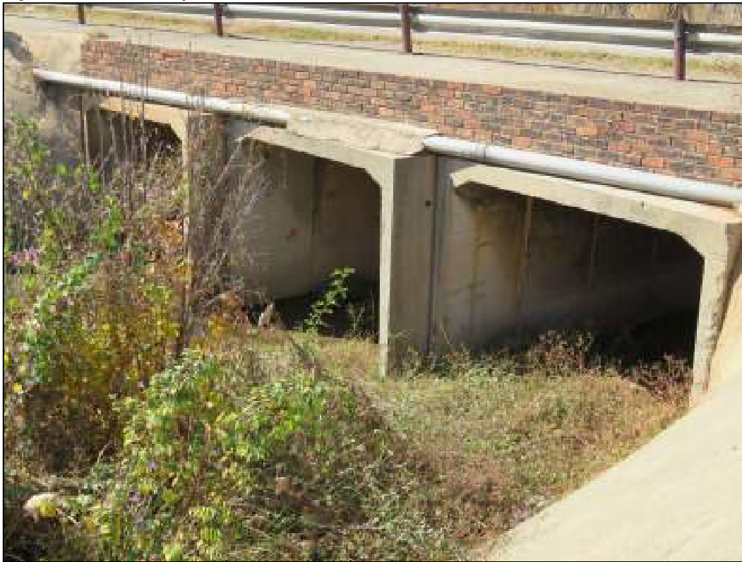
Figure 7-3 Percy Sherwell street culvert
