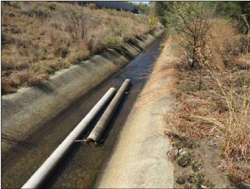
Figure 7-4 Downstream concrete, parabolic channel
