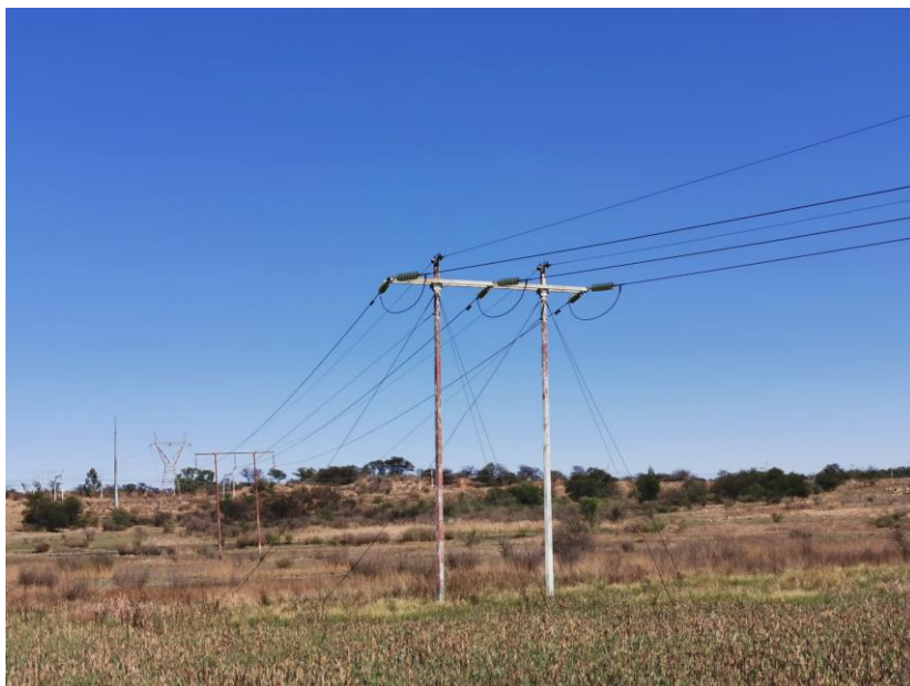
Fig 1.3 – Existing 88kV Incomer to Sonland Milan Substation
