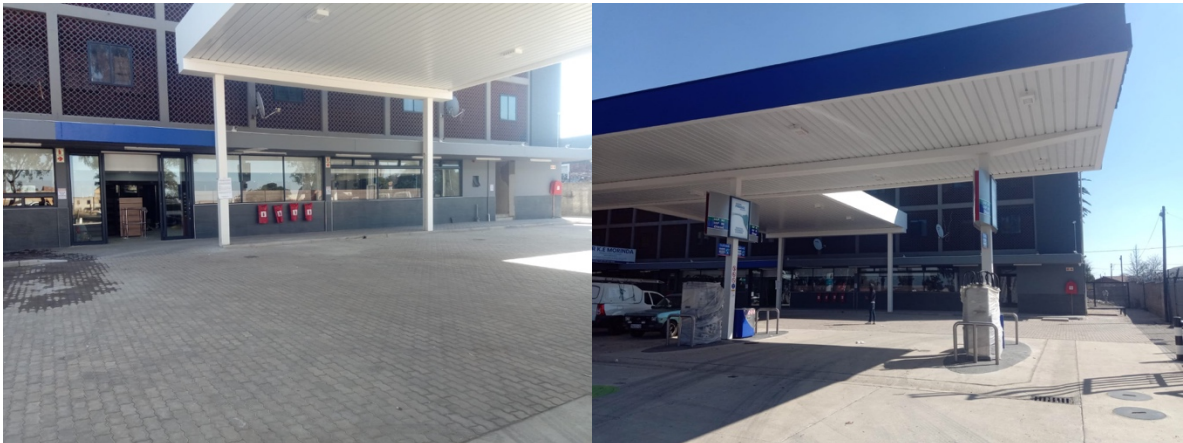
Close-up view from the R29, W.
