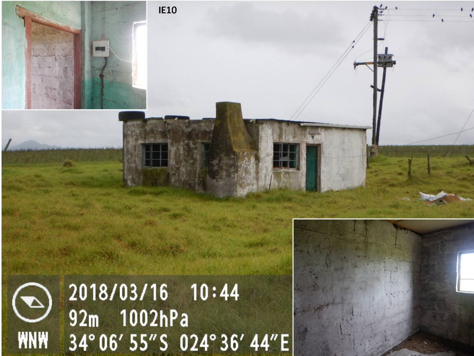
Plate 7. Non conservation worthy historic period structure with mixture of clay and cast cement bricks, not directly impacted by proposed development.
