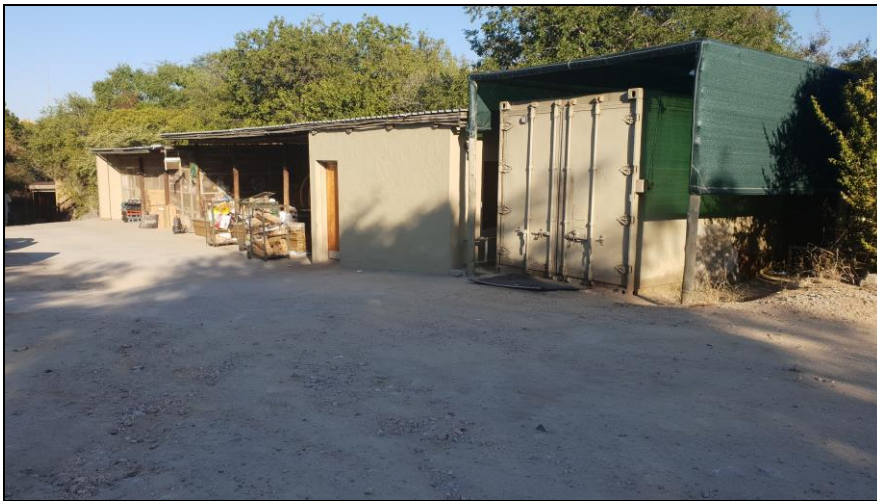
Figure 12: Existing infrastructure at the lodge
