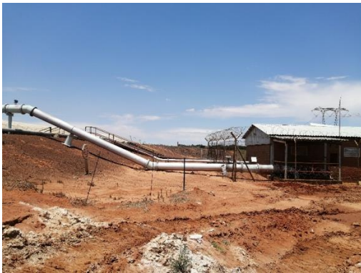
Figure 7 - Eastern view of Dam pump house.
