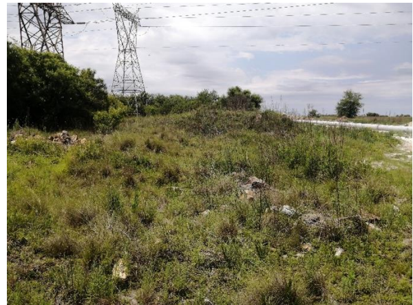
Figure 8 - Dumping occurring along the East Pump Station pipeline.
