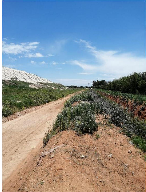
Figure 6 - Eastern view of Moab Khotsong Sewage Works pipeline
