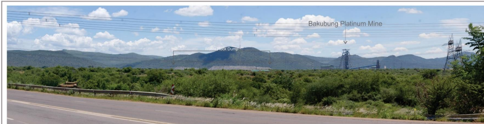
View 3a: From a Elandriver Bridge (R565), approximately 0.7km south-west of the proposed TSF site.
