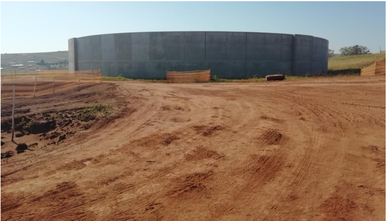
Plate 1: Photo 1: View of reservoir where pipeline will connect(Photograph © by Author 2019).
