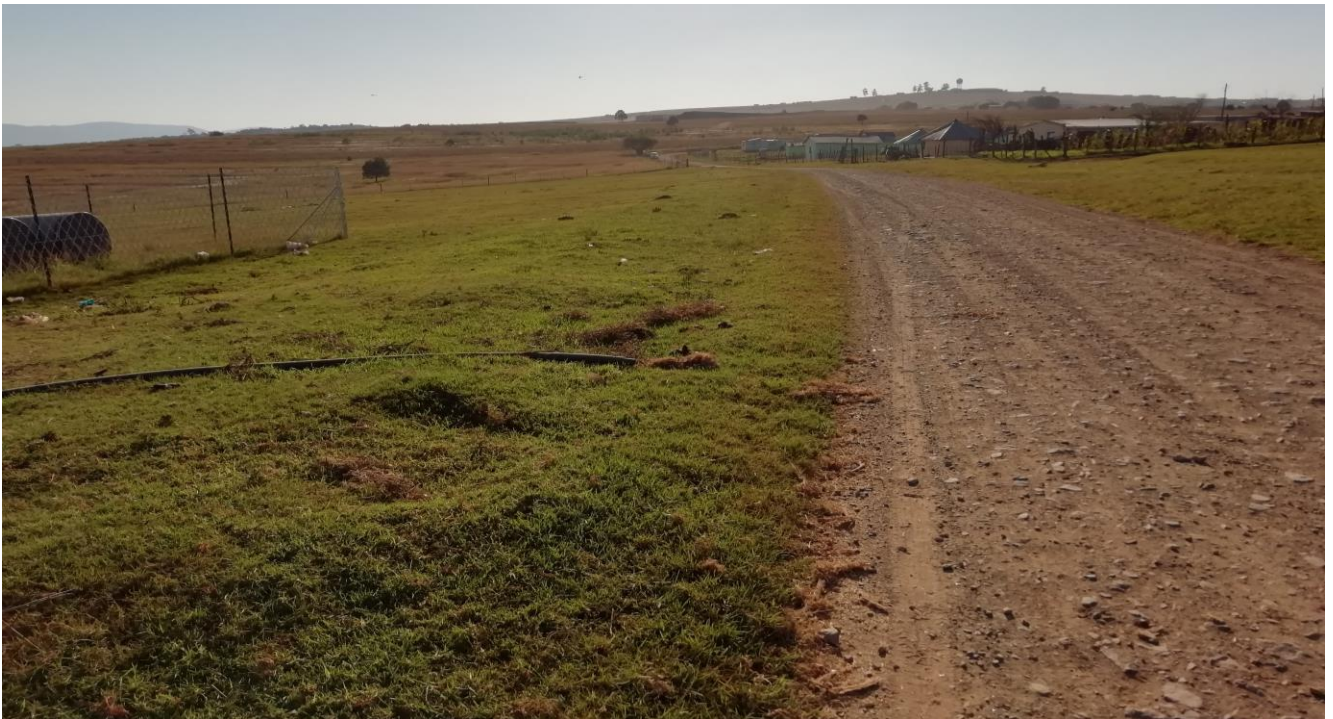
Plate 3: Photo 3: View of access road to the pipeline route and Rosedale Water works (Photograph © by Author 2019).
