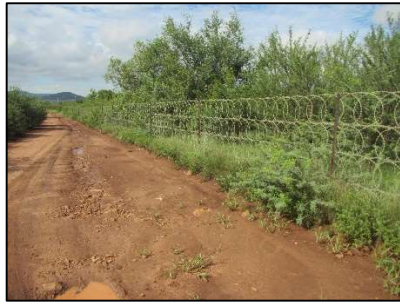
Figure 6: Gravel access road and razor-wire boundary fence
