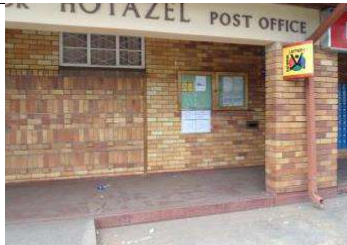
Site notice 7: Hotazel Post Office
