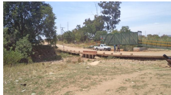
Figure 4: 2013 Downstream Site B1 was dry during the November site visit.
