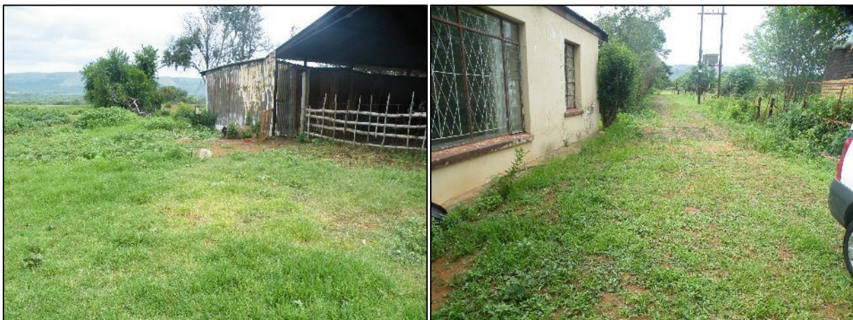
Photograph 2: Infrastructure north of the R560
