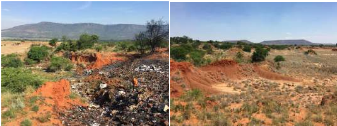
Figure 11: Waste material being deposited between the donga valleys (left). On the right is donga erosion exposing deeply (3-4m deep) incised and weathered in-situ soil. Donga erosion is on the southern fence boundary portion of the landfill where dumping is yet to reach.
