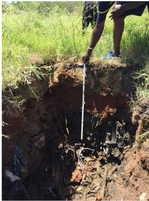
Figure 14: STP4 test pit profile showing capping soil over waste.
