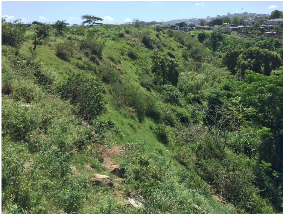
Figure 8: Vegetated landfill slope looking northwestwards.
