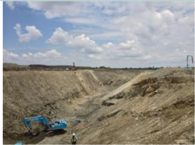
Although the open pit will be moderately intrusive in the visual landscape, its physical extent at any given time will be limited
