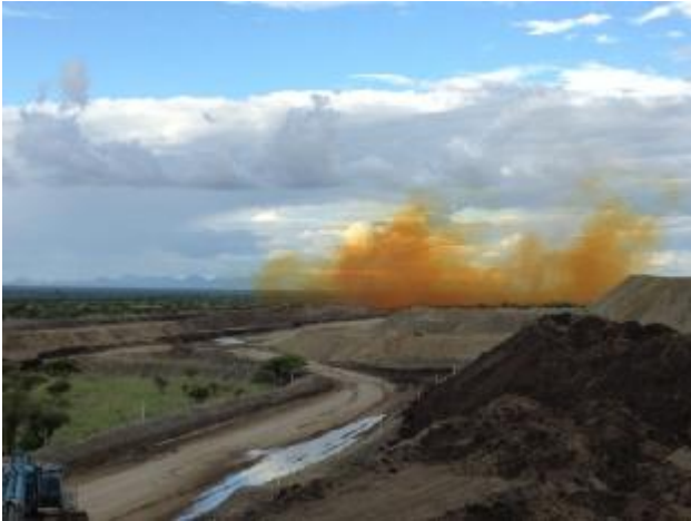
Airborne dust can be particularly bothersome and more visible than its cause and will result in moderate visual intrusion
