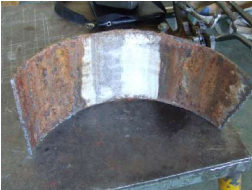
Section cut off from a 520mm diameter steel pipe which recently failed. Corrosion inside the pipe is severe with no evidence of any concrete lining remaining. Wall thickness of the pipe is less than 2mm in the vicinity of the longitudinal weld.
