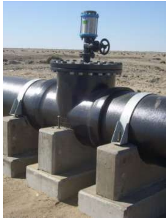
Typical Above Ground Installation of a 600mm diameter pipeline and air-valve arrangement
