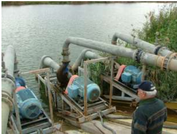
Typical examples of pumps on a trolley configuration
