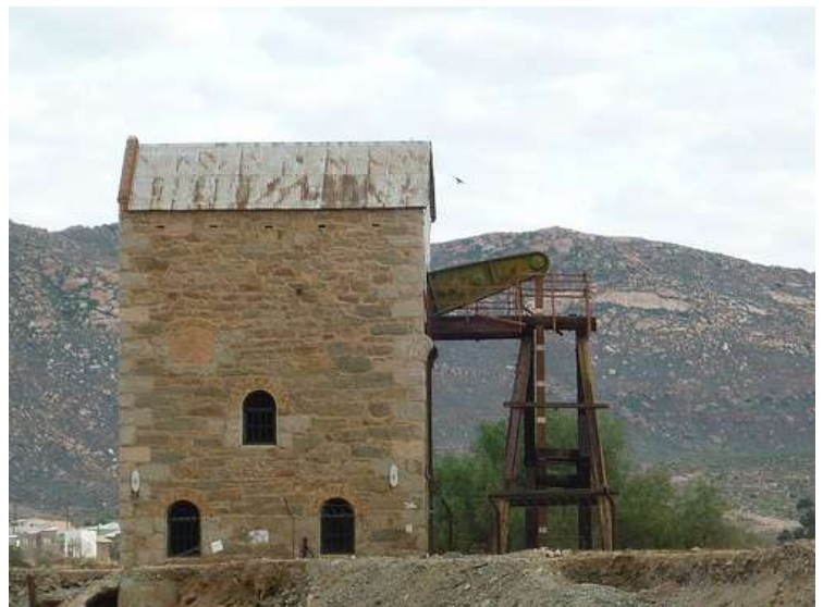
Remains of a Cornish Beam Pump in Okiep
