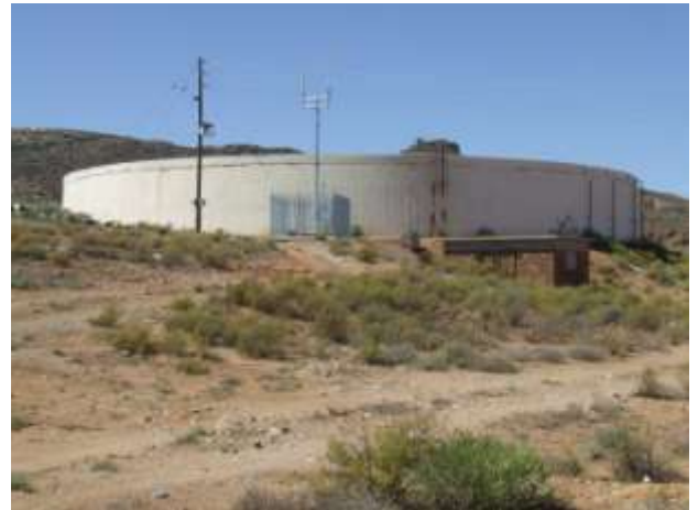
Vaalhoek Reservoir near Okiep
