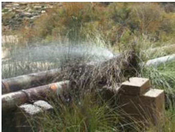
Typical leaks and failures occurring on the NababEEP gravity mains
