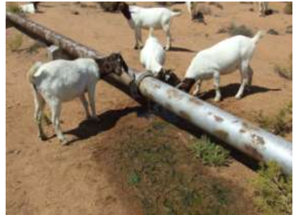
Leaks on the Okiep – Garagoup steel rising mains
