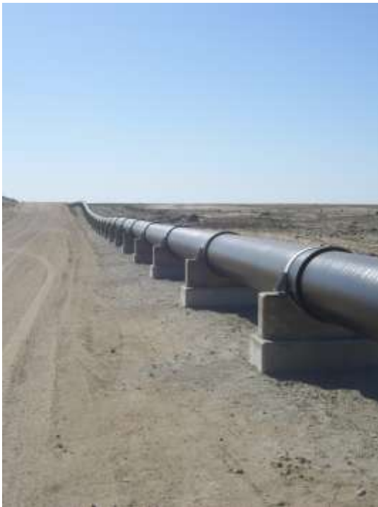
Typical Above Ground Installation of a 600mm diameter pipeline and air-valve arrangement
