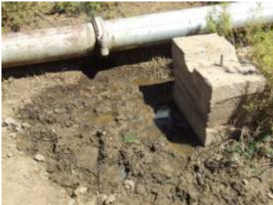
Leaks on the Okiep – Garagoup steel rising mains
