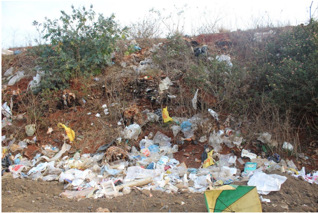
Figure 3: Historical 'end-tipping' method of landfilling noted on rehabilitated section of the landfill
