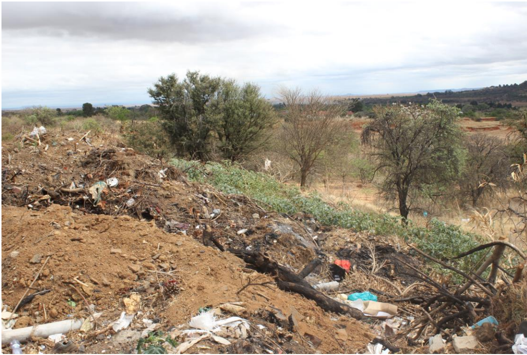
Figure 3: Historical 'end-tipping' method of landfilling noted on eastern active section of the landfill
