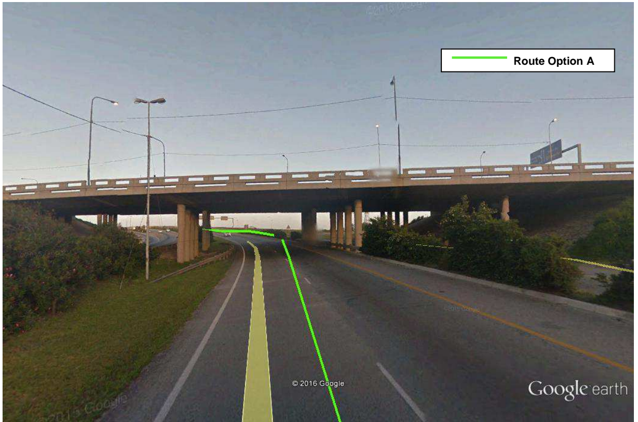
Google Image 8: “Street View” of the N2 National Freeway crossing the Settlers Way (M4) Bridge. This non-avoidable bridge has a soffit clearance height limitation of only 5.05m. This will have an influence on the type of transport trucks, which should be made available.
