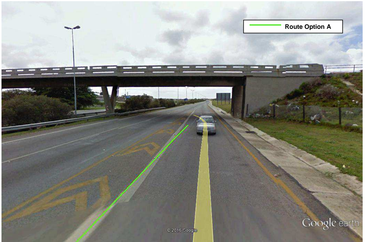
Google Image 10 : “Street View” N2 National Freeway crossing Cradle Road Bridge. This bridge has a soffit height clearance of 5,18m. No transport problems are foreseen.
