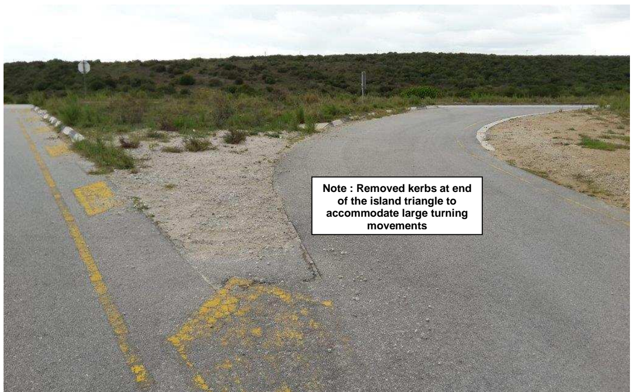
Photos 6 (above) and 7 (below) : View of the intersection and slip road at the R367 / R334 (Daniel Pienaar Road). A traffic island with raised barrier kerbs is situated within the transport vehicle movement. Some of the kerbs of this island have previously been removed (not yet replaced) to make provision of large abnormal turning movements. This may be sufficient or minor additional modifications and minor earthworks and vegetation clearance may still be required. Roadside furniture (eg. signposts and poles) may have to be temporary removed / permanently be relocated to accommodate the sweep path of the transport vehicles.
