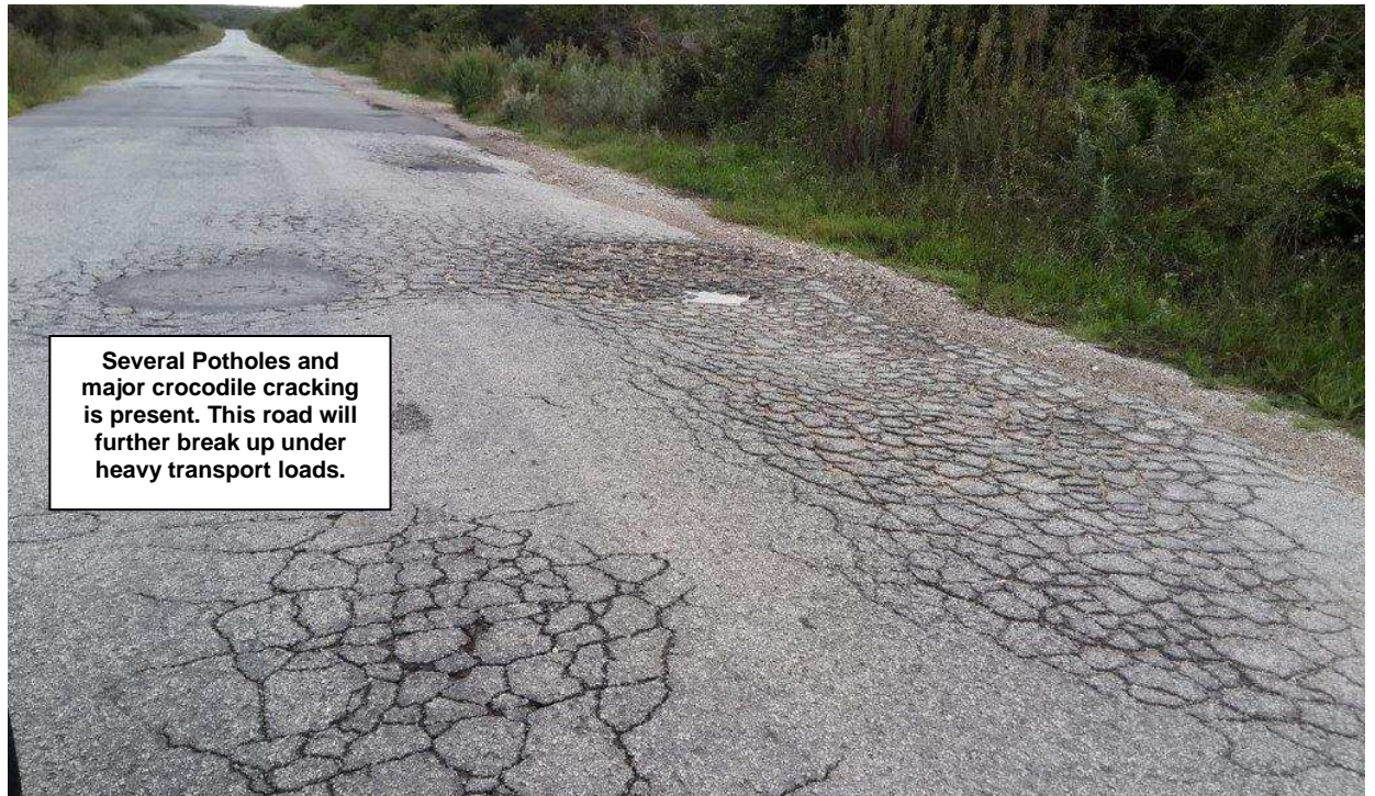
Photos 10 (above) and 11 (below): The condition of Daniel Pienaar Road (R334) between the R367 (R102) and the R335 intersection is poor / not desirable with a large extent of crocodile cracking, potholes and pavement failures are present. The road section will require minor rehabilitation to safely accommodate transport vehicles.
