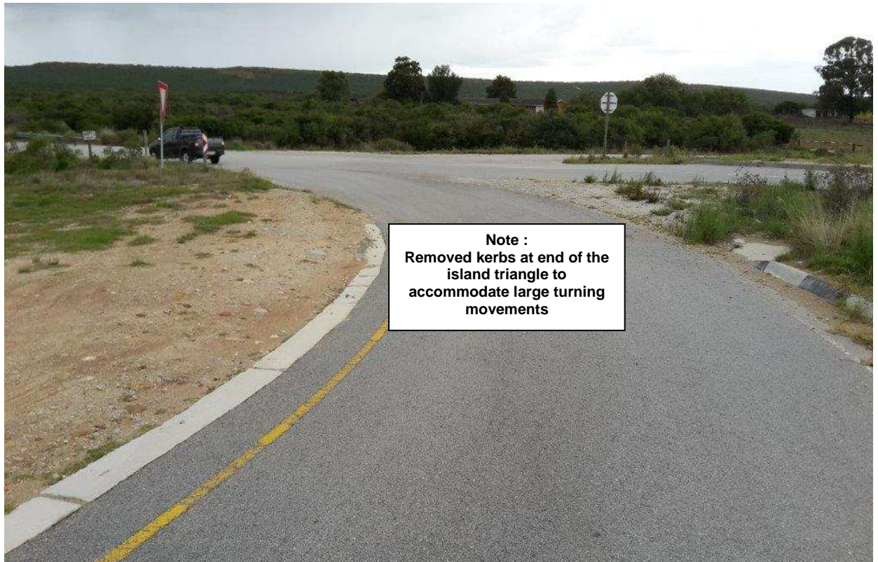
Photos 6 (above) and 7 (below) : View of the intersection and slip road at the R367 / R334 (Daniel Pienaar Road). A traffic island with raised barrier kerbs is situated within the transport vehicle movement. Some of the kerbs of this island have previously been removed (not yet replaced) to make provision of large abnormal turning movements. This may be sufficient or minor additional modifications and minor earthworks and vegetation clearance may still be required. Roadside furniture (eg. signposts and poles) may have to be temporary removed / permanently be relocated to accommodate the sweep path of the transport vehicles.
