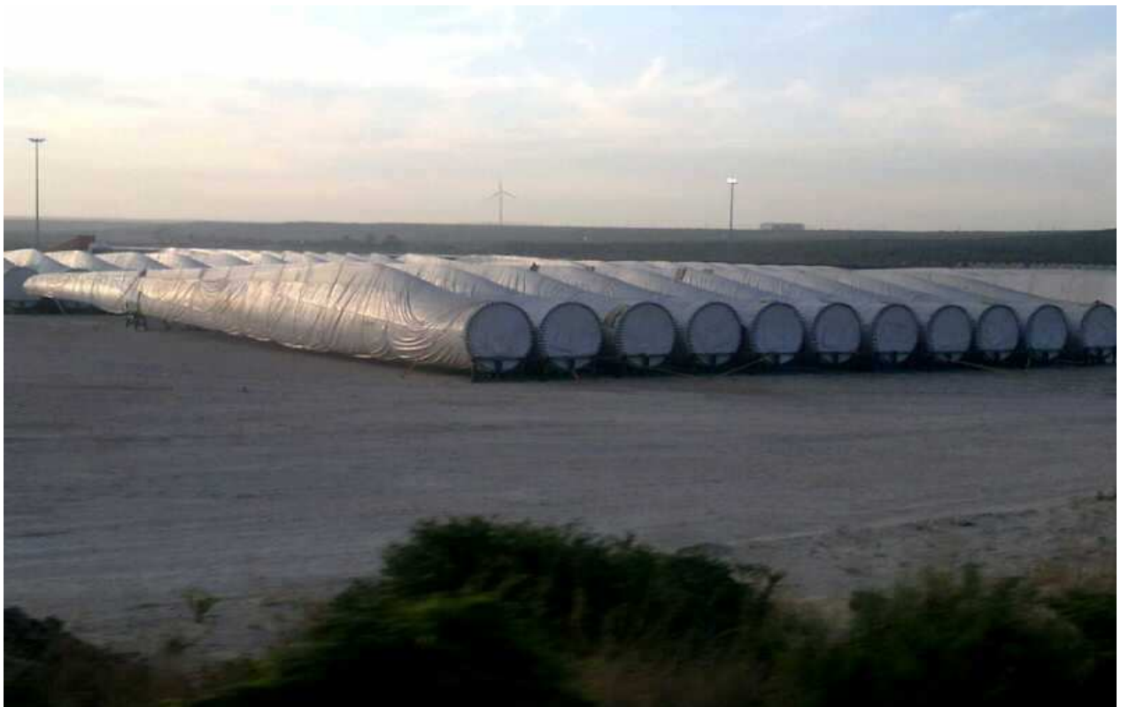
Photo 12 : View of typical turbine blade laydown area – note large open (hard surface) spaces required to safely manoeuvre the abnormal trucks and mobile cranes in and around the turbine laydown area.
