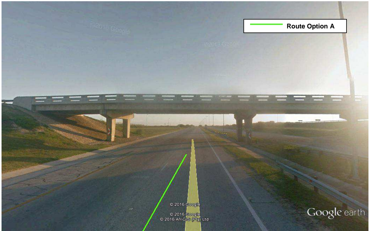
Google Image 4: "Street View" N2 National Freeway crossing the R335 Bridge.
