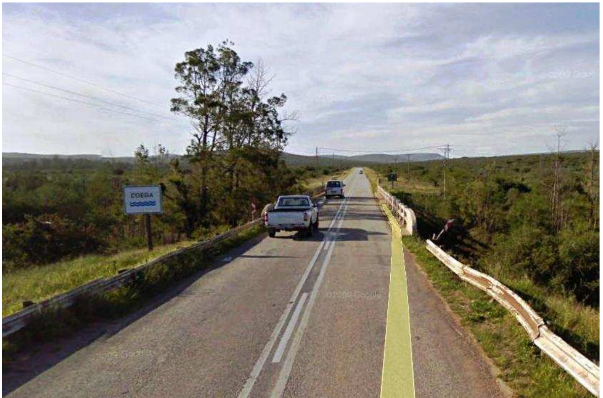
Photo 16 : View of the narrow Coega River Bridge – full road closure of this section of the R75 will be required
