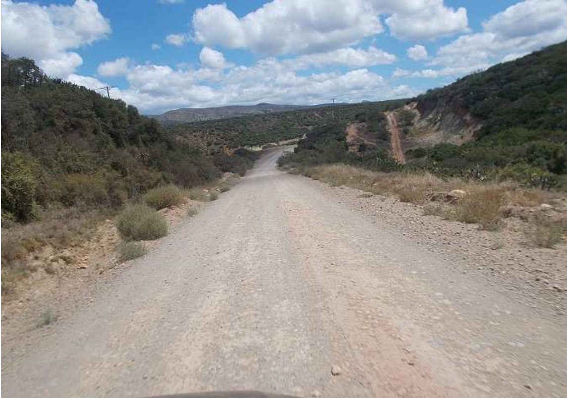
Photo 21: A number of noticeable horizontal and vertical curves (crests and sags) are located along this route. These areas will need to be surveyed and assessed during Detail Design stage which may require reshaping of the road.
