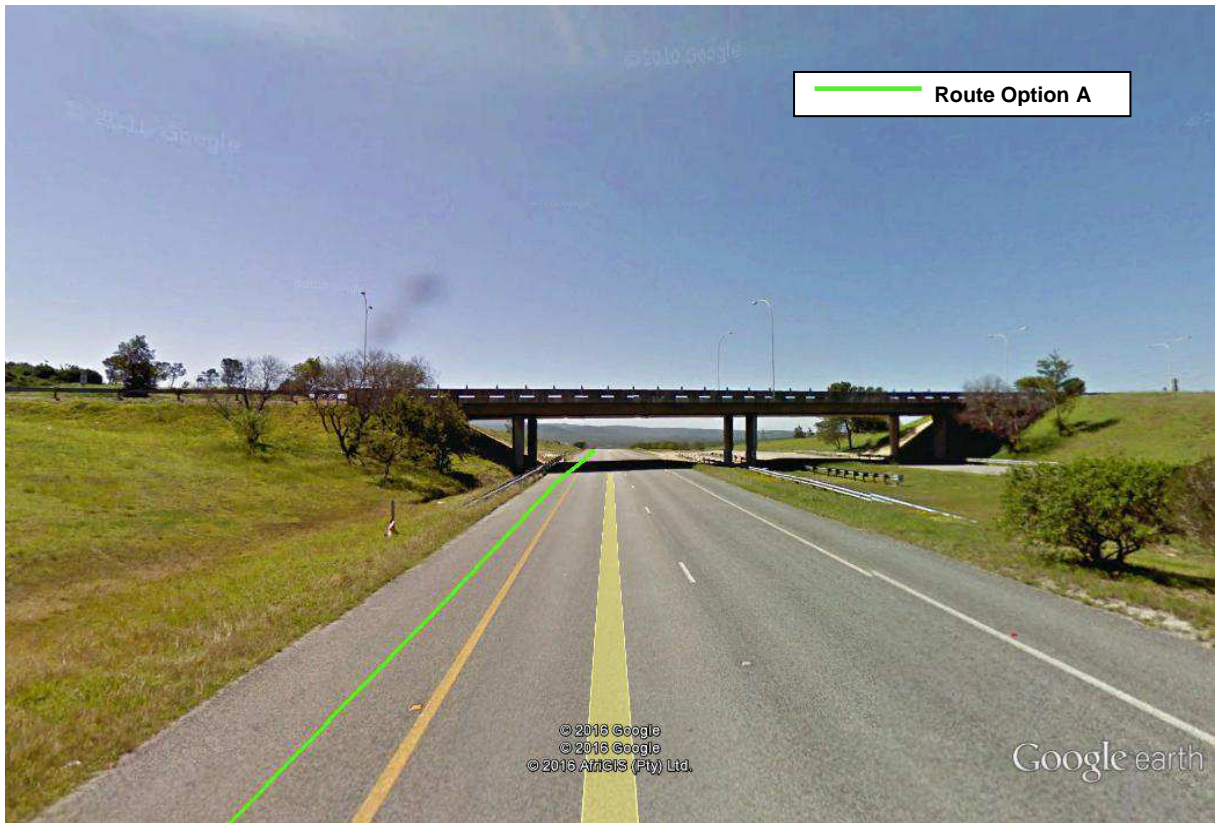
Google Image 16: "Street View" R75 crossing Botha Road Bridge.
