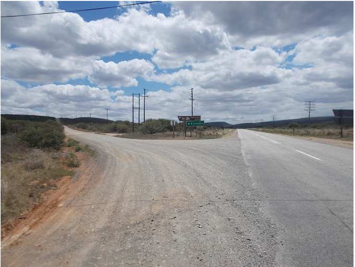
Photo 19: Y-junction R75 / MR407 intersection. No road widening or removal of any roadside furniture is envisaged.
