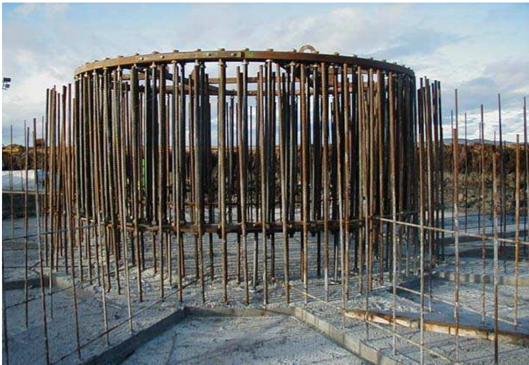
Photo 1a and 1b: Siemens Foundation Anchor Ring Assembly
