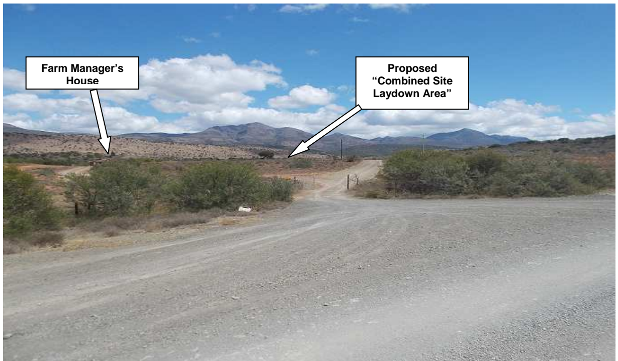
Photo 23: View of the entrance to the Roodeplaat Wind Farm Development site from the MR407 Provincial Road to Minor Road MN50474 and “Combined Laydown Area” in the background. This intersection will be widened to accommodate the turning radii of transportation vehicles. The work will entail minor earthworks and removal of bushes, boundary fences and the existing gate.
