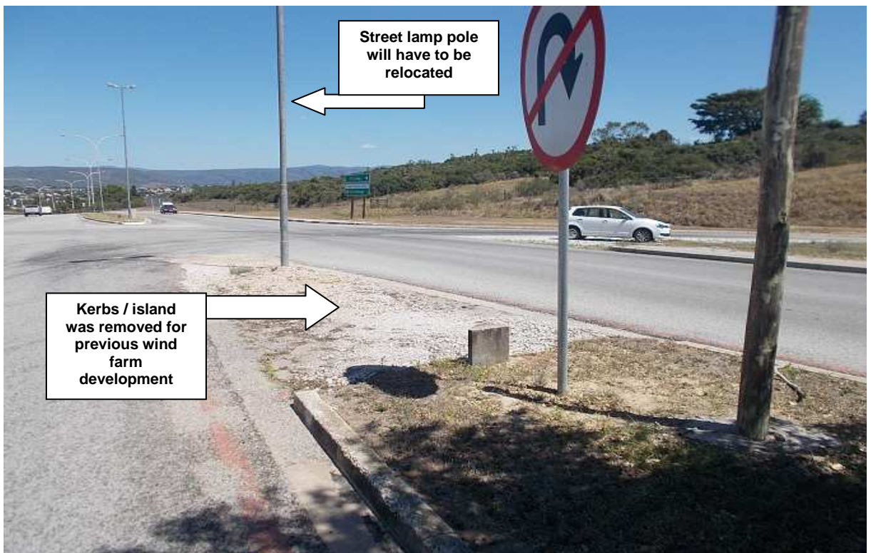
Photo 14: Adequate turning radii may not be available at this R75 on-ramp. However it is possible to temporarily widen the road through removing additional the inside kerbs. Minor earthworks may be required. Roadside furniture (signposts, traffic control signs etc.) including the street lights will have to be temporarily removed / permanently relocated to accommodate the sweep path of the transport vehicles.
