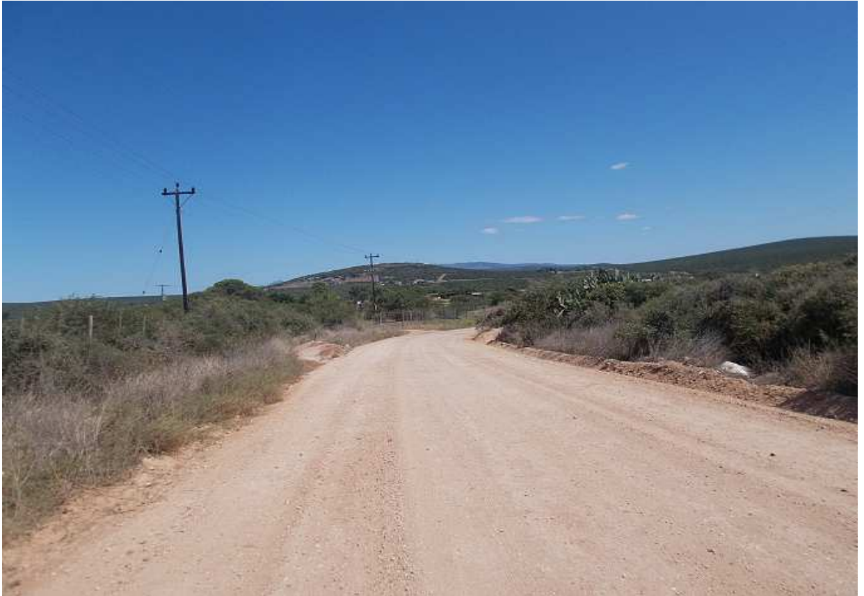
Photo 16: Noticeable horizontal and vertical crest/sag curves are situated along this road. These areas will need to be surveyed and assessed at detail design stage.
