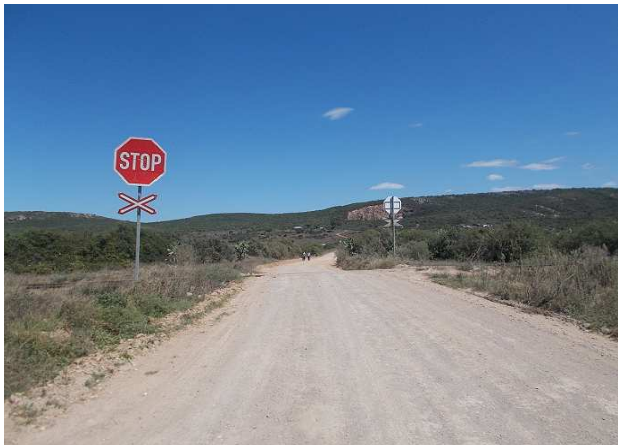
Photo 17: A railway level crossing may need to be upgraded to accommodate transportation vehicles.
