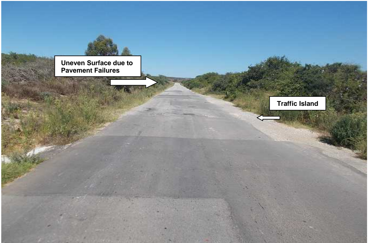
Photos 8 (above) and 9 (below): The condition of Daniel Pienaar Road (R334) between the R367 (R102) and the R335 intersection is poor / not desirable with a large extent of rough pothole plugging and pavement failures are present. The road section will require minor rehabilitation to safely accommodate transport vehicles.
