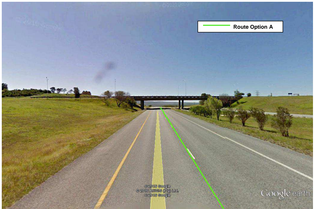
Google Image 18: "Street View" R75 crossing the R334 Bridge. Sufficient soffit clearance for more than 5,5m is available. No problems are foreseen.
