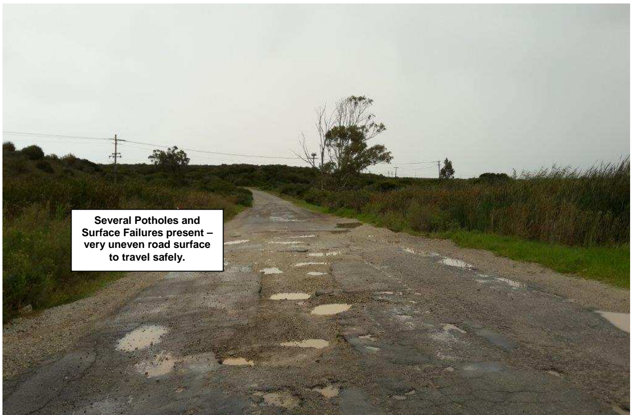
Photos 10 (above) and 11 (below): The condition of Daniel Pienaar Road (R334) between the R367 (R102) and the R335 intersection is poor / not desirable with a large extent of crocodile cracking, potholes and pavement failures are present. The road section will require minor rehabilitation to safely accommodate transport vehicles.
