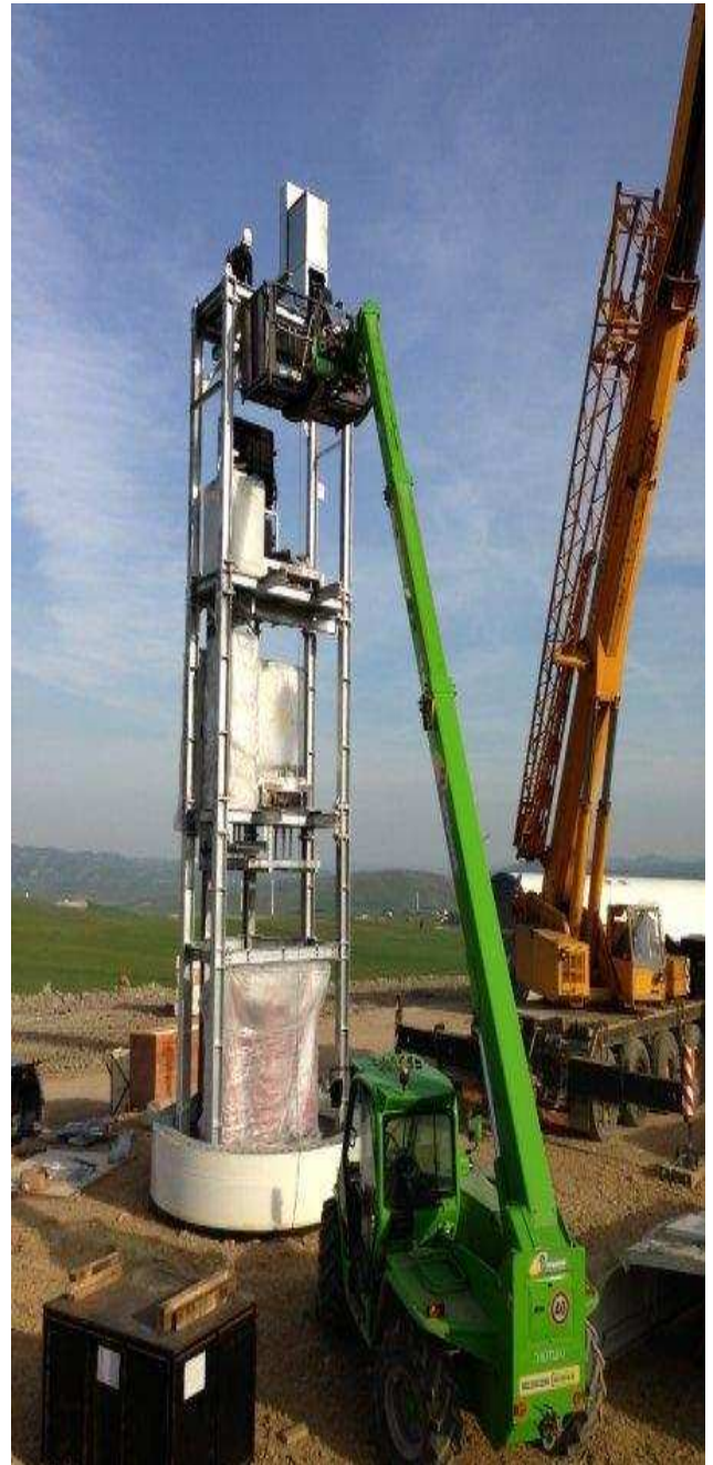
Photo 13 & 14 : Typical Mobile (self-driven) and Primary Fixed (lattice boom type) cranes which will have to be available at each Turbine Platform area, during the turbine erection process.
