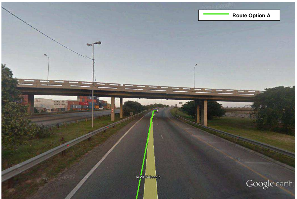
Google Image 9: “Street View” N2 National Freeway crossing the Kempston Road Bridge.
