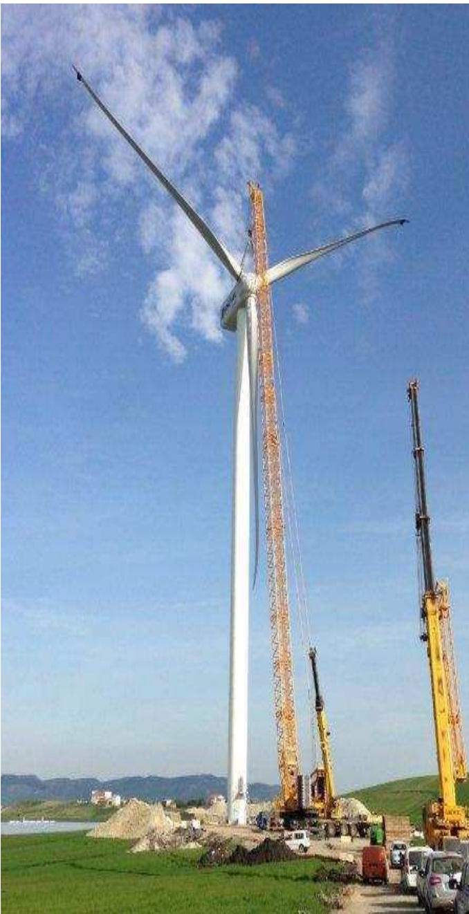
Photo 13 & 14 : Typical Mobile (self-driven) and Primary Fixed (lattice boom type) cranes which will have to be available at each Turbine Platform area, during the turbine erection process.
