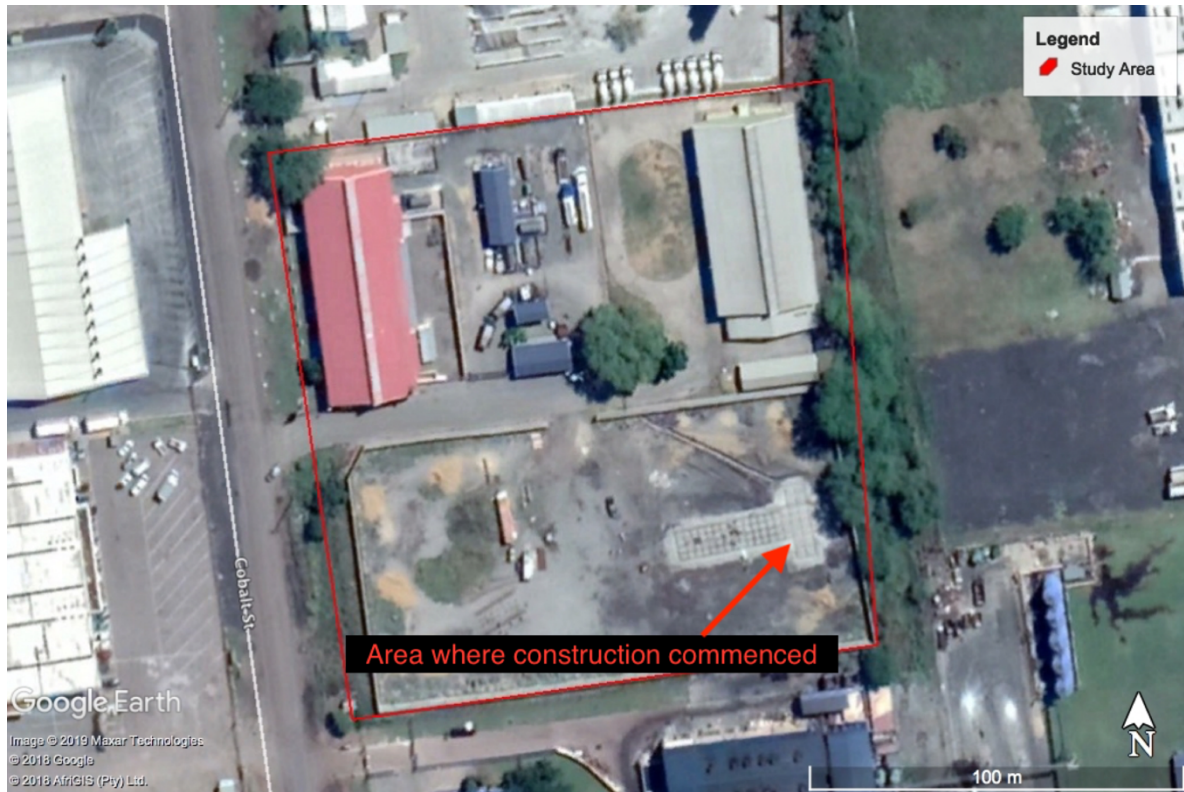
Figure 5: Activities commenced with: bunded area to the east, and pillars of canopy in area east-west
