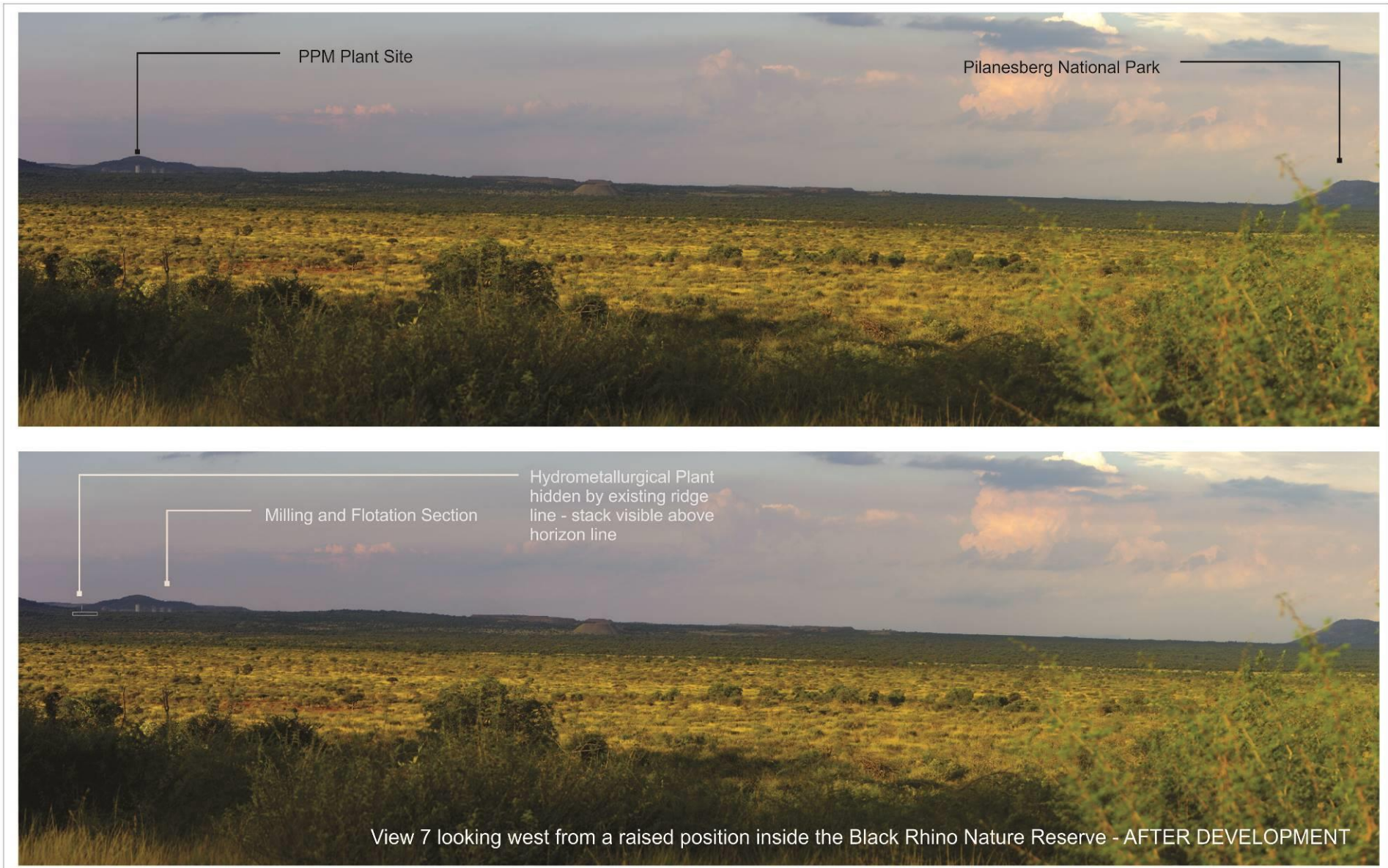
Figure 15: SIMULATION View 7 - PPM Plant Expansion Project
