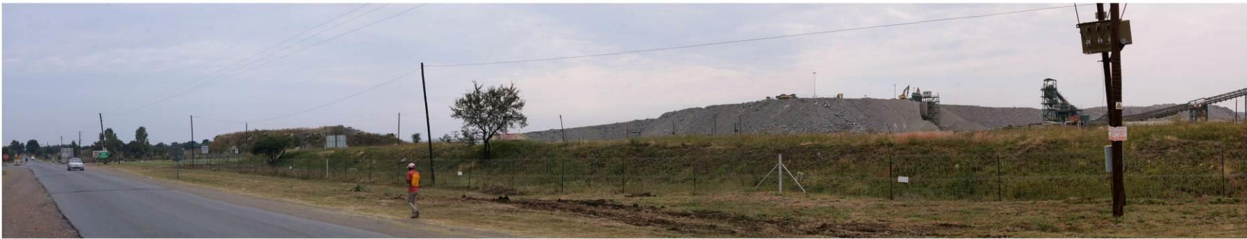
View 6a: View towards the Tharisa Platinum Mine mining infrastructure
