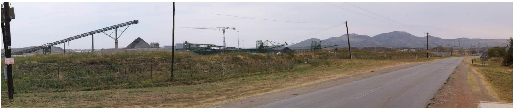
View 6b: View towards the Tharisa Platinum Mine mining infrastructure
