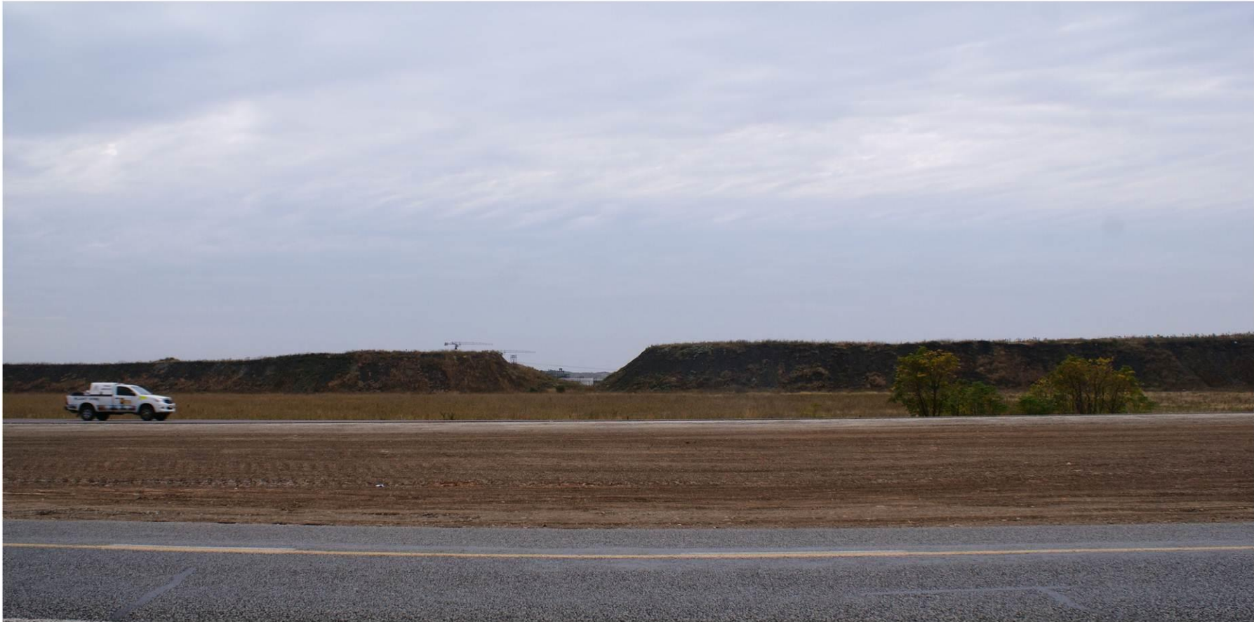
View 8: View from the N4 towards the Tharisa Platinum Mine, mining infrastructure visible through the gap in the berm
