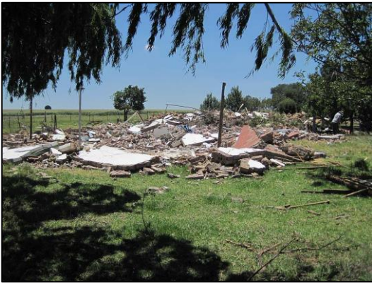
Figure 12 – Rubble from demolished house
