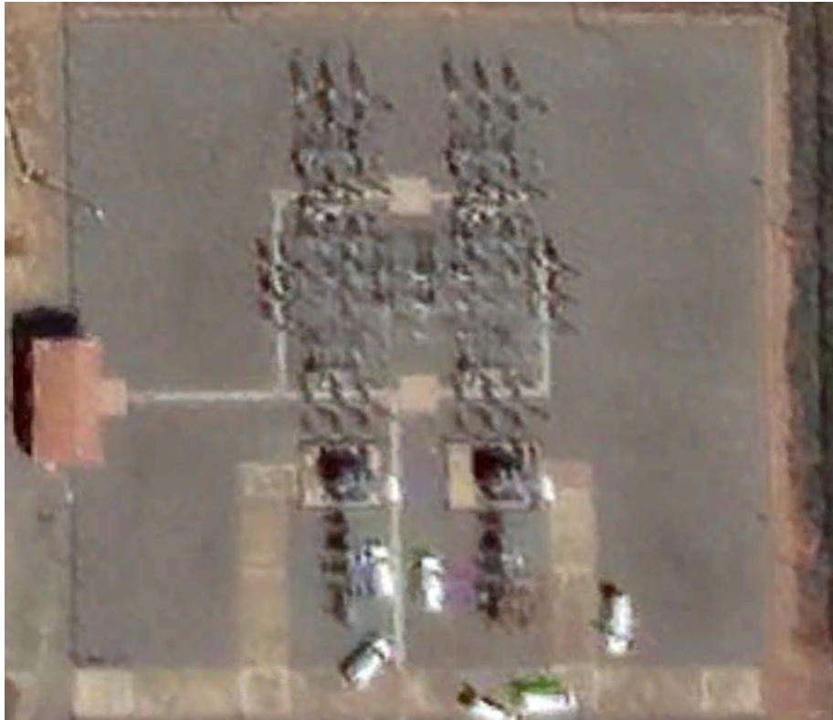
Figure 4: Google Earth Picture of Joel Substation
