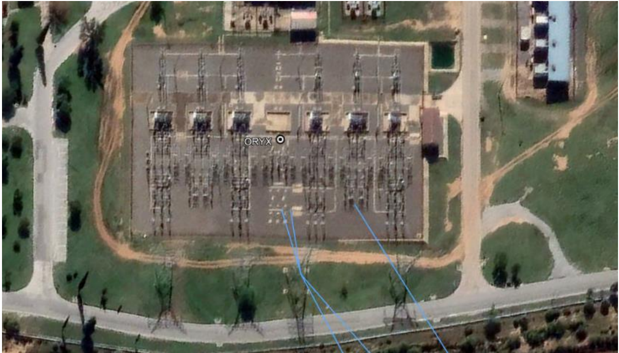
Figure 6: Oryx Substation Google Earth Picture
