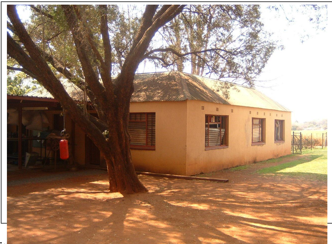
Figure 8- A historical house (HC01.3) which is part of Historical Complex 01 (above). The original rectangular core of the house was extended with several rooms. The house (core) was constructed during the 1860's.
