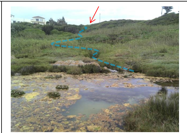
Photo 2: Area 1 – Channel formed as a result of the stormwater outlet (indicated by the red arrow).
