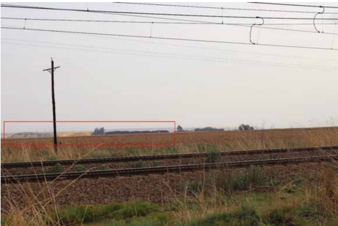
Figure 19: Potential Future View from Viewpoint 4 in a Southerly Direction towards the Project
