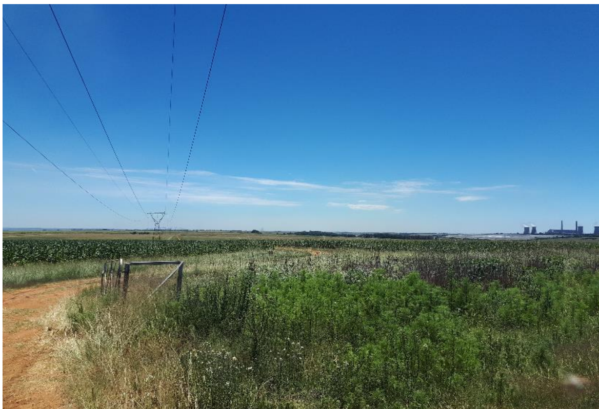
Figure 25: View west from dirt road toward Arnot Power Station (RHS) and Alternative 1 and 2 sites (LHS) with 132kV power line visible traversing both Alternative 1 and Alternative 2 sites.
