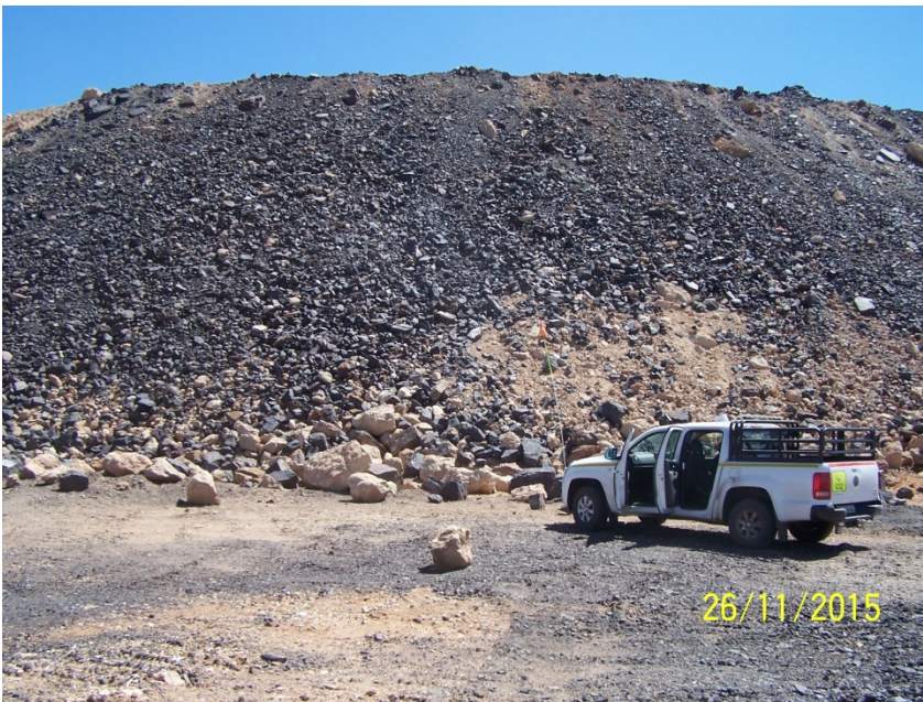
Figure B5: Side slopes of Western dump, mixture of shale and calcrete
