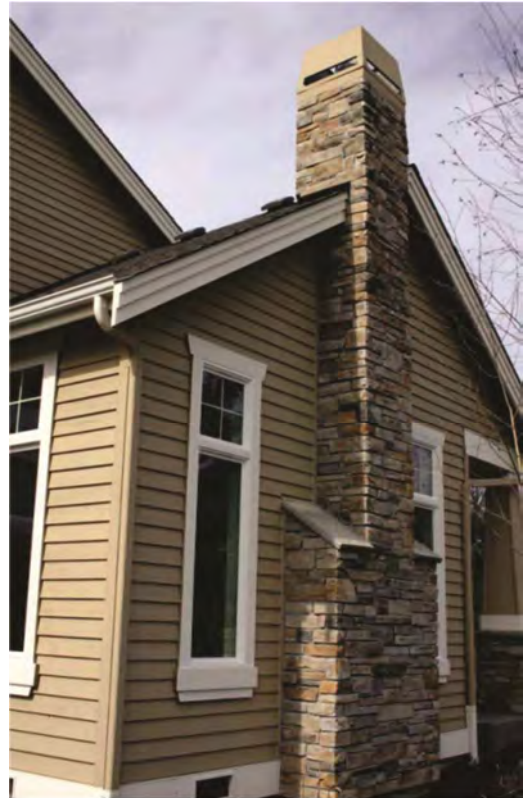
An example of a stone chimney and ship-lap cladding
