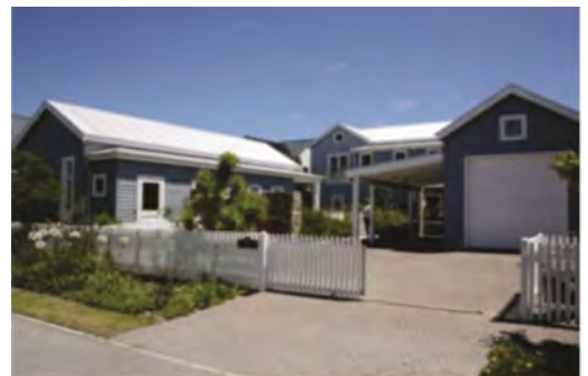
External walls in a combination of smooth plaster surface and Nutec ship-lap boarding.
