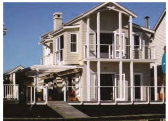
White powder coated aluminium window & door frames and white timber detailing
