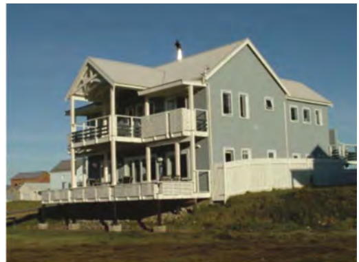
Double pitched roof of approximately 35° with gable end
