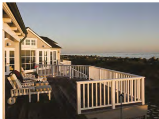
Generous timber deck with simple, elegant, white-painted timber balustrading
