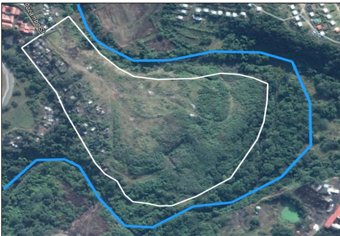
Figure 5: Shakaville Landfill Aerial Image (2013)
