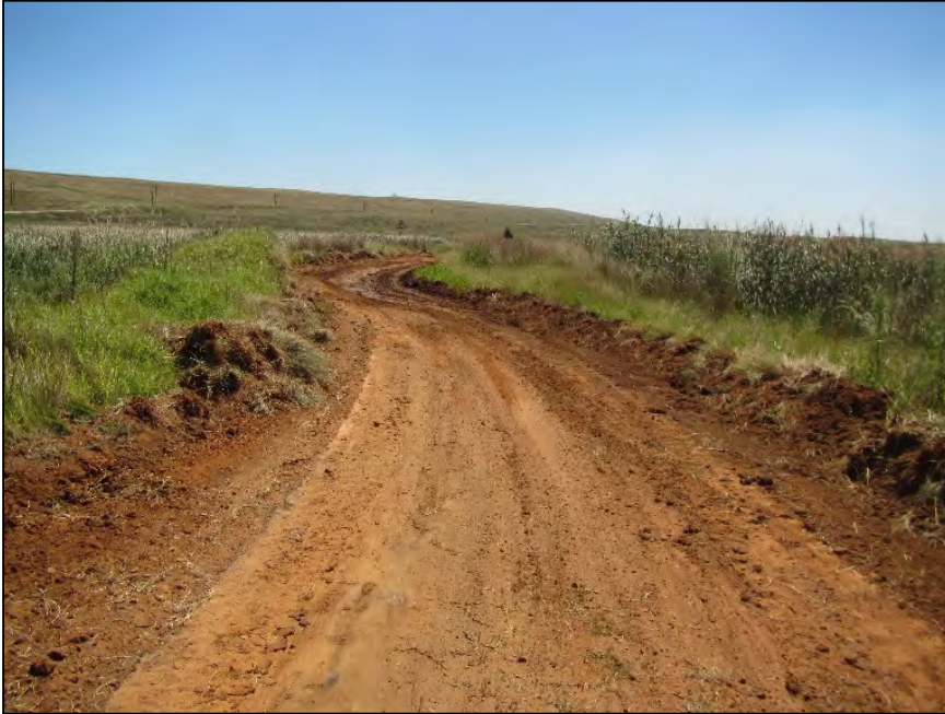
Figure 14: Existing road traversing an area of wetland
