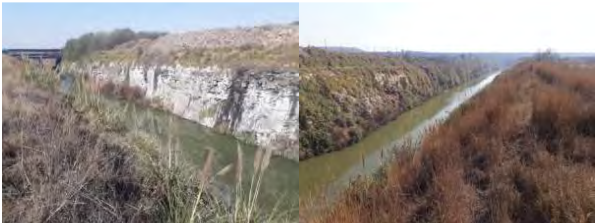
Figure 10. Photographs of the Steenkoolspruit River diversion to the west of the South Pit study area.
