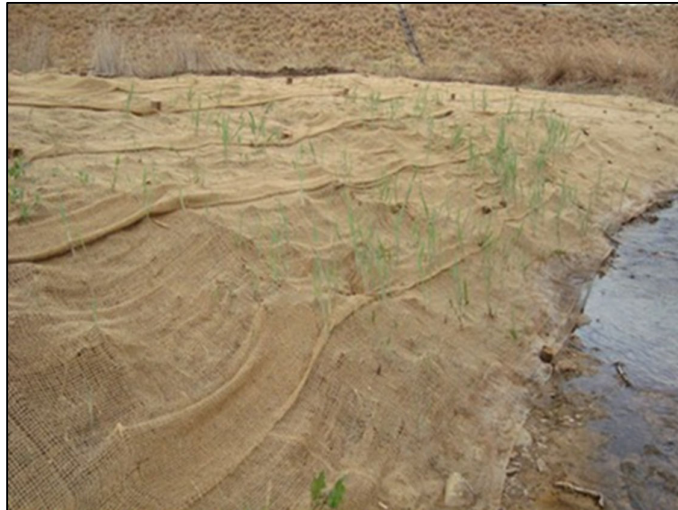
Figure 10: Geotextile used for re-seeding
