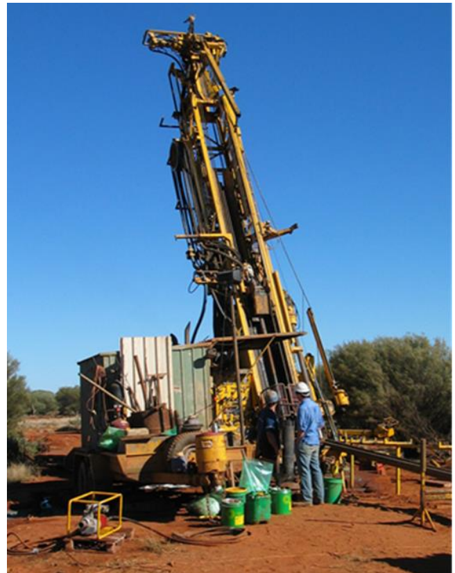
Figure 3: Example of well drilling operations
