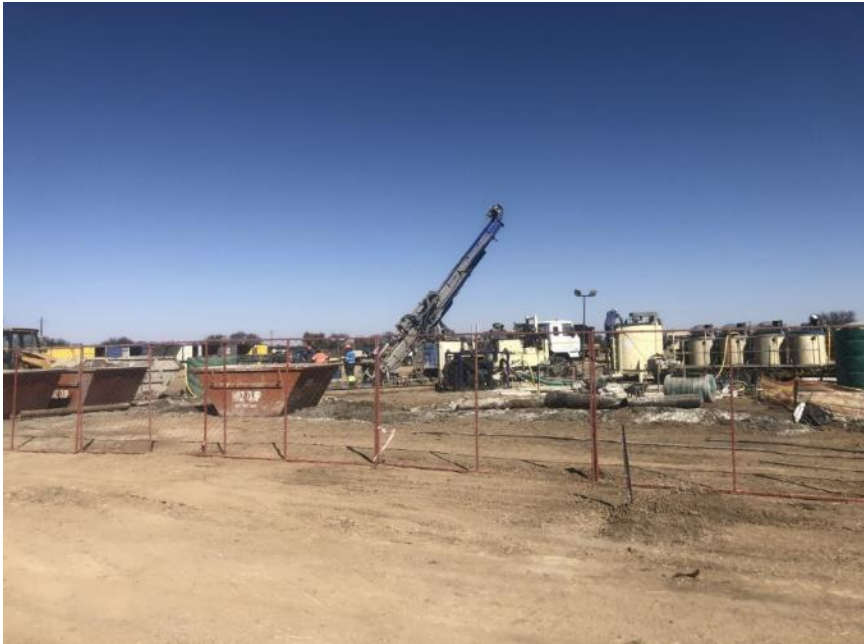
PLATE 16, DRILLING OPERATIONS UNDERWAY DURING PHASE 1 EXPLORATION
