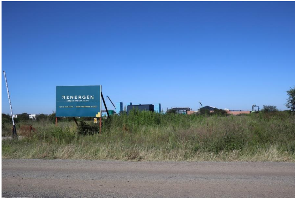
PLATE 7 – EXISTING PHASE 1 TETRA 4 COMBINED HELIUM AND LIQUID NATURAL GAS PLANT
