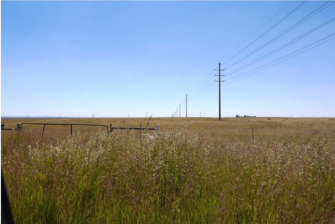
PLATE 20 - A VIEW ALONG THE LINE OF A 132KV OVERHEAD POWER LINE WITH MONOPOLE TOWERS
