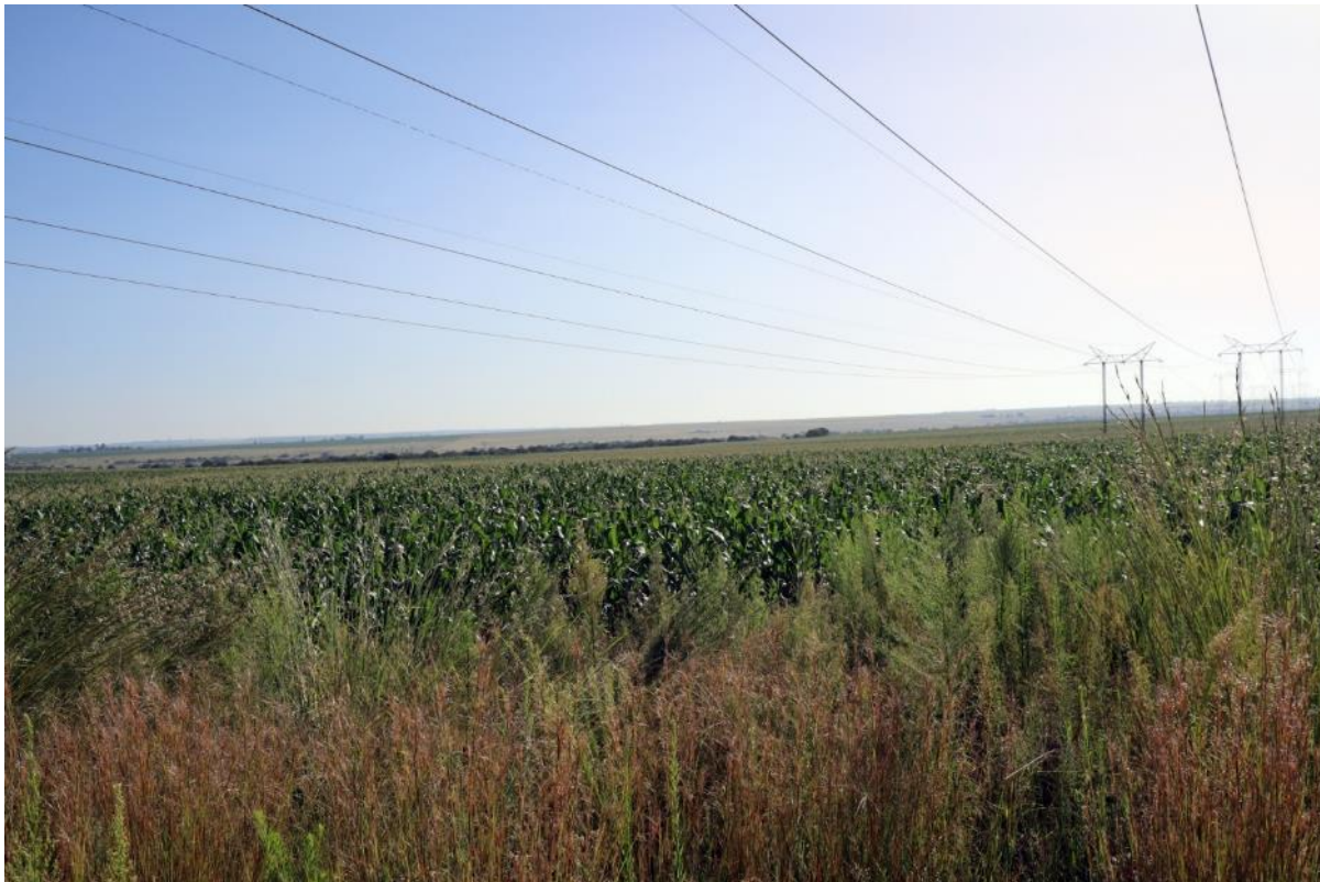
PLATE 25, VIEW OF THE EXISTING EVEREST PERSEUS 275KV OVERHEAD POWER LINE FROM THE R30
