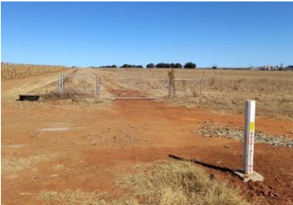
PLATE 3 – TYPICAL PIPELINE SERVITUDE
