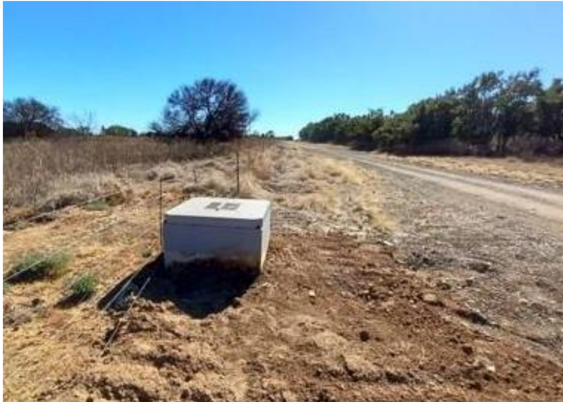
PLATE 4 – LOW POINT DRAIN
