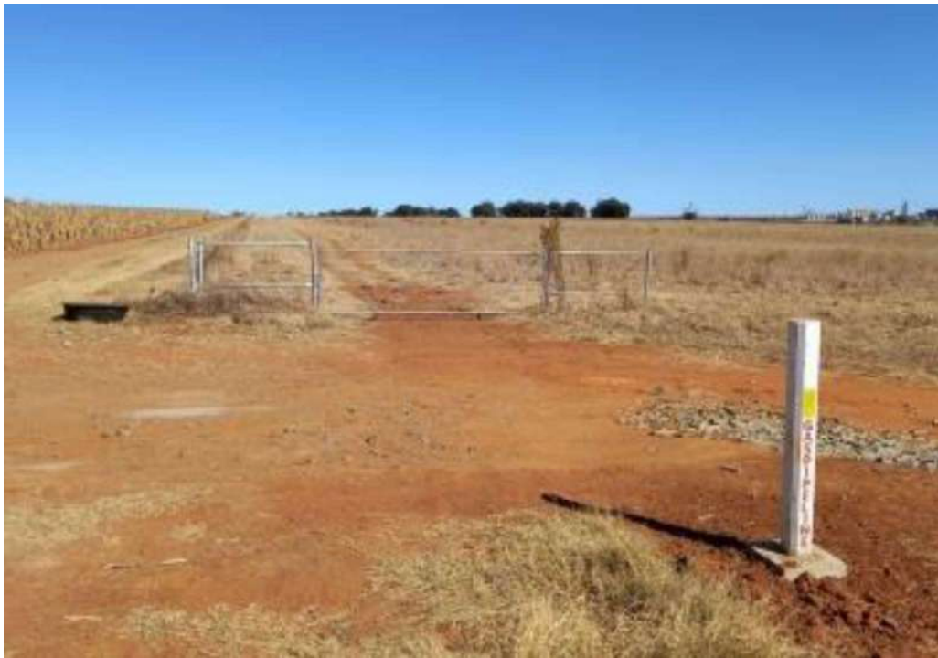
Figure 8: Typical pipeline servitude and pipe marker.
