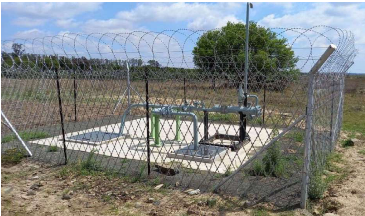
Figure 9: View of an existing pigging station constructed as part of Cluster 1.
