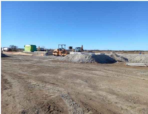
Figure 17: Typical example of helium / LNG Plant construction.
