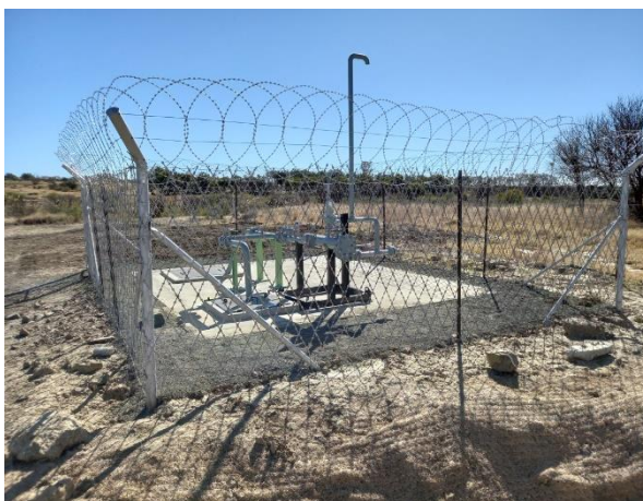
Figure 13: Pigging Station.
