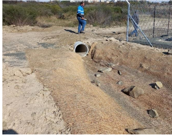
Figure 16: Typical example of access road flume pipe.
