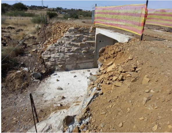
Figure 15: Typical example of culvert on access road.
