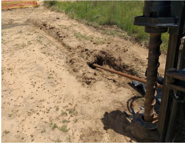
Figure 9: Typical example of exploration drilling.
